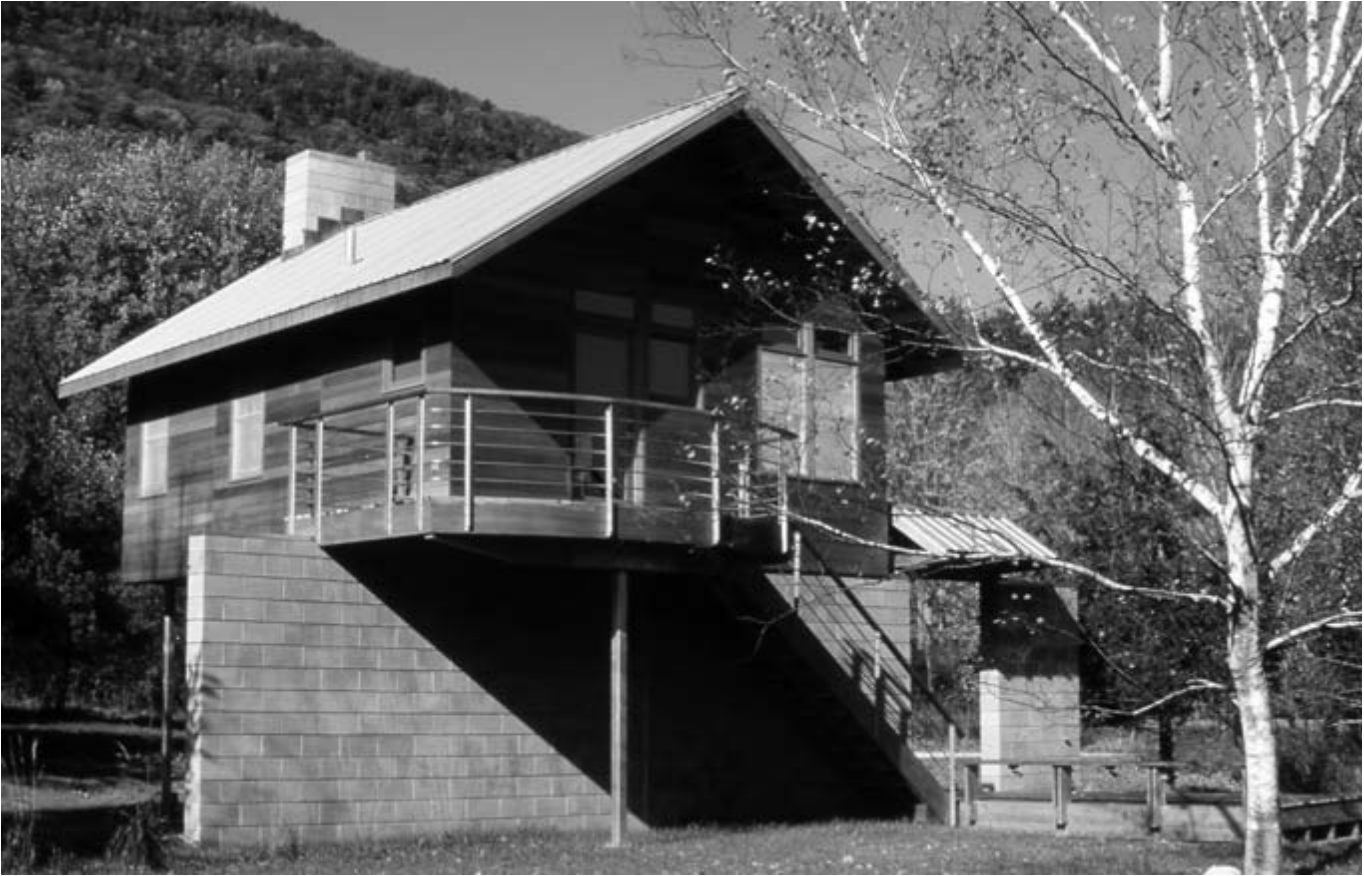
FIGURE 3-1. A CONCRETE BLOCK WALL ANCHORS THE HOUSE TO THE SITE AND ALIGNS IT WITH THE CARDINAL DIRECTIONS. HOUSE FOR TWO ARTISTS, THE BERKSHIRES, MASSACHUSETTS
