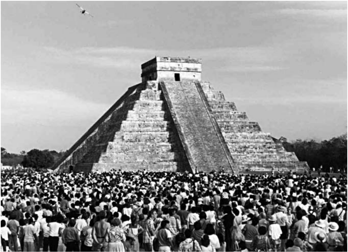
FIGURE 12-2. THE GREAT PLAZA OF CHICHÉN ITZÁ CAN COMFORTABLY ACCOMMODATE THE MORE THAN THIRTY THOUSAND VISITORS WHO ATTEND THE DESCENT OF THE "SERPENT OF LIGHT" ALONG THE BALUSTRADE OF THE MAIN CASTILLO PYRAMID EACH SPRING EQUINOX. SUCH ARCHITECTURAL SPACES WERE SITES OF THE CEREMONIAL EVENTS CHARACTERISTIC OF THE THEATRIC MODE.
