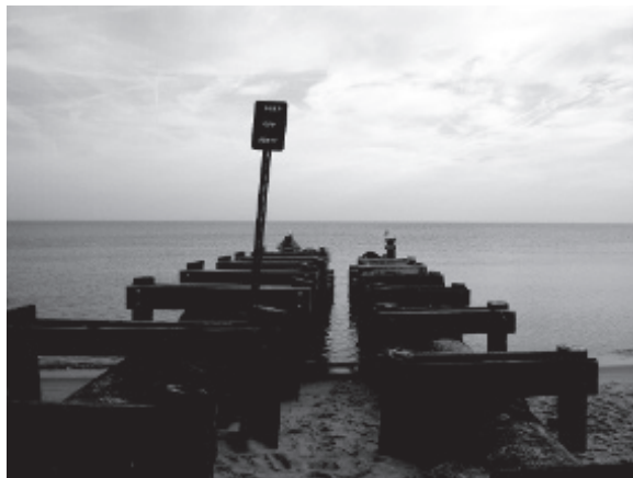
FIGURE 10.11 Stormwater outfall pipes at Ocean View Beach, Chesapeake Bay, Norfolk, Virginia. (Photograph by F.R. Spellman.)
