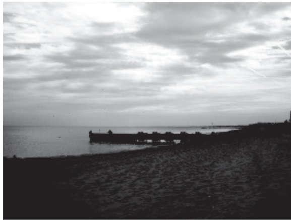
FIGURE 10.10 Stormwater outfalls at Ocean View Beach, Chesapeake Bay, Norfolk, Virginia. (Photograph by F.R. Spellman.)
