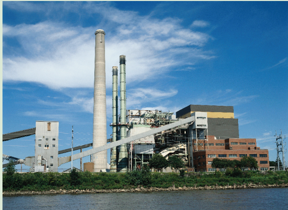
Ohio Edison plants provide electrical service to more than 1 million customers. © Don Farrall/PhotoDisc/Getty Images.
