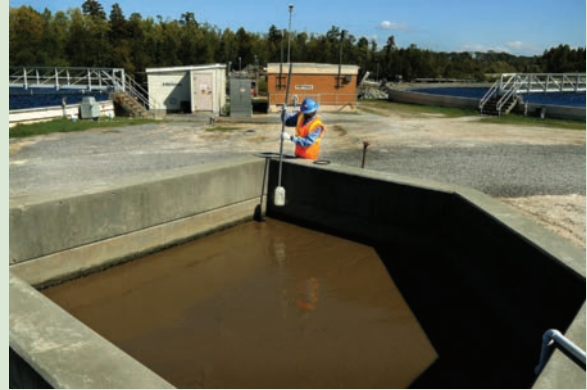
Effluent at this facility must fall within a statistically determined pH range. © ZUMA Wire Service/Alamy Limited.
