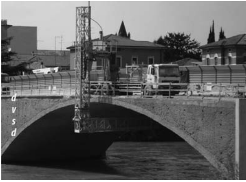
Figure 9. Hydro-demolition at the intrados of the arches of the S. Francesco Bridge.
