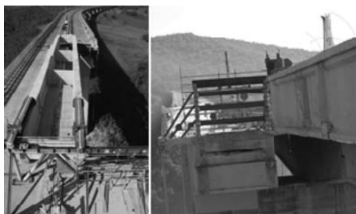
Figure 1. Shifted grid and first beam ready for demolition.
