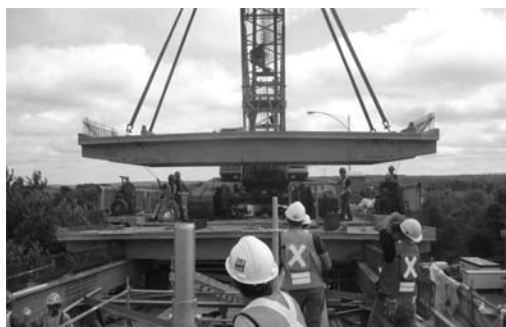
Figure 1. Deck panel installation.
