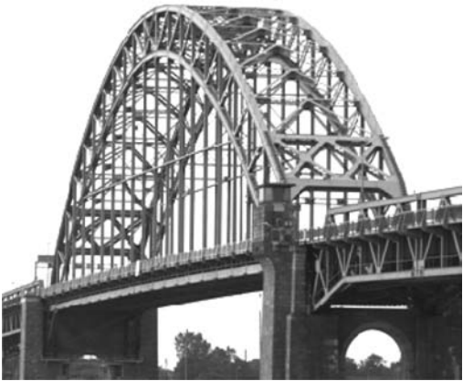
Figure 1. TPB Steel Tied Arch Span.
