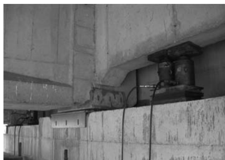
Figure 1. Lifting system and new bearing under construction.
