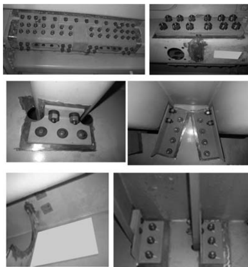
Photo 3. Repair of fatigue cracks.
