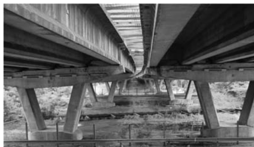
Figure 1. Example of a beam and slab bridge (VIPP bridge), the Merlebach bridge.
