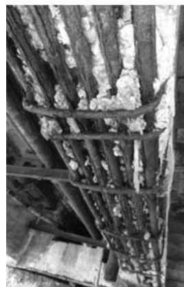
Figure 2. Damage due to steel corrosion on the longitudinal edge girders.
