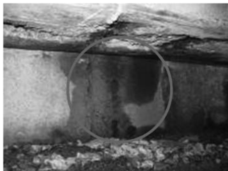
Figure 1. Water leakage from expansion joints.
