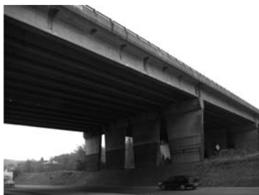
Figure 1. Example of a VIPP bridge.
