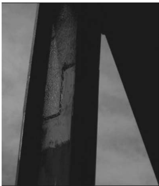
Figure 11. Repair executed in the broken post in the Correntes River Bridge.
