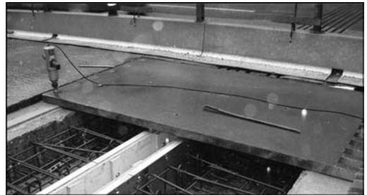
Figure 3. Installation of TensaFlex sliding finger joint “under traffic” using Mini-Fly-Over traffic management system.
