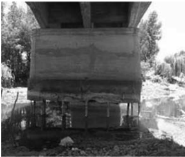
Figure 1. Scour and erosion in San Luis bridge.
