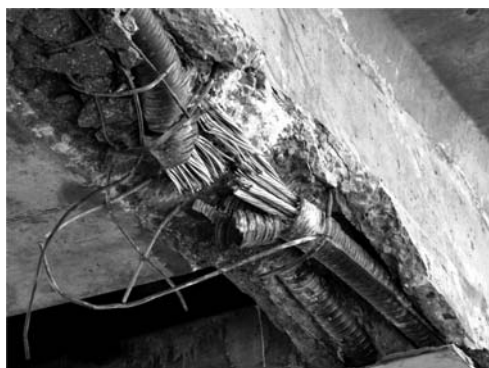
Figure 1. Extent of damage to web and tendons.
