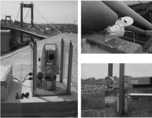
Figure 2. RTS unit on control room roof and reflectors on Saltash tower (top right) and Plymouth side tower (bottom right).
