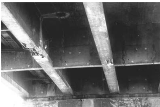
Figure 3. Damages at the bottom flanges of VIPP beams due to poor waterproofing.
