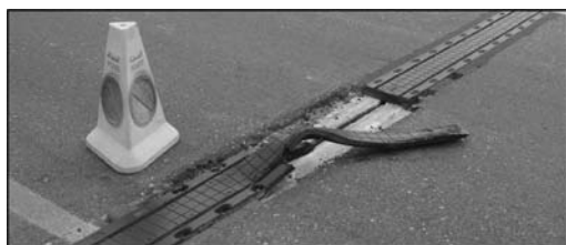
Figure 1. A low-quality, small movement expansion joint in urgent need of replacement.
