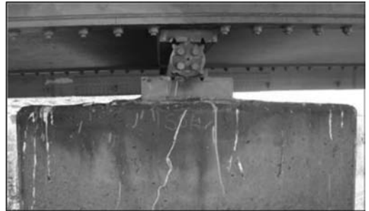
Figure 2. Typical roller bearing.
