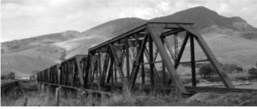
Figure 5. View of the Doce II River Bridge showing the six spans with a total length of 247.60 m.
