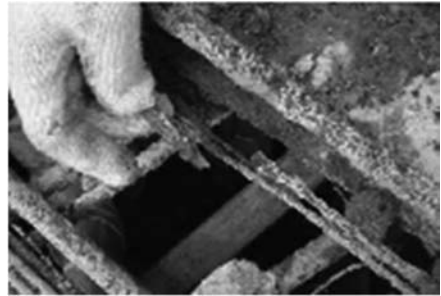
Figure 1. The situation of the broken prestressing strands in the deck slab.
