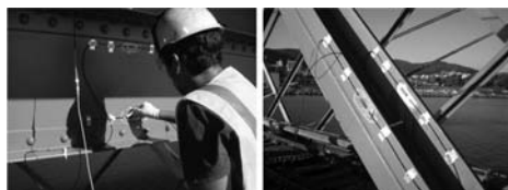
Figure 2. FBG strain sensors installation.
