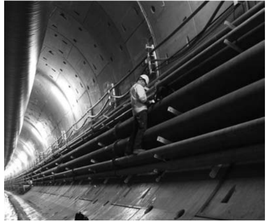
Figure 1. Downloading of strain measurement data in the Liefkenshoek Tunnel.
