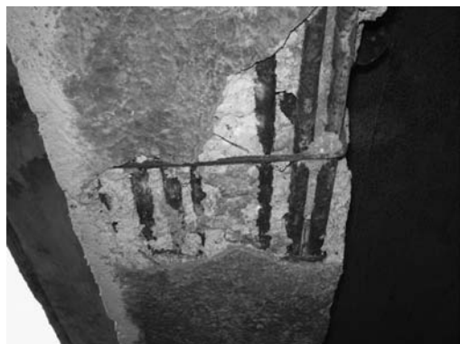
Figure 1. Example bridge with spalling of the concrete cover.
