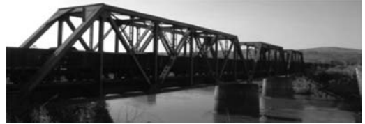
Figure 4. View of the Doce I River Bridge showing the three Warren truss spans with a total length of 103.10 m.
