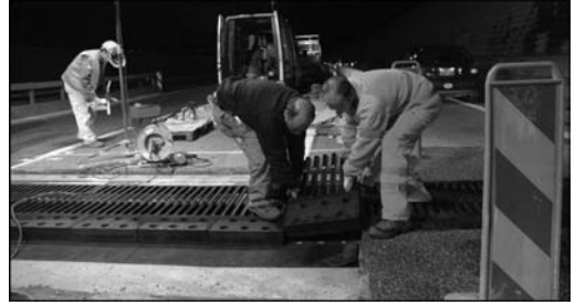
Figure 2. Installation of TensaFlex sliding finger joint.
