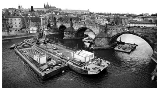
Figure 1. Deepening of pillar fundaments.
