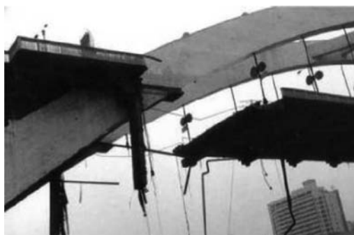
Figure 1. Short suspenders collapsed of Nanmen Bridge in Sichuan, China.
