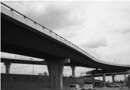
Figure 1. Steel trapezoidal box girder bridge at US 290 E and IH 35 in Austin, TX.
