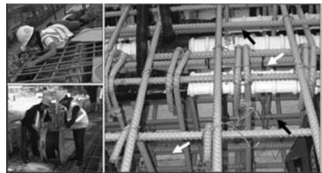
Figure 2. Photographs taken during sensor installation. Top left: Student installing sensor. Bottom left: Students installing extension cable. Right: Parallel discrete and distributed sensors installed on rebar.
