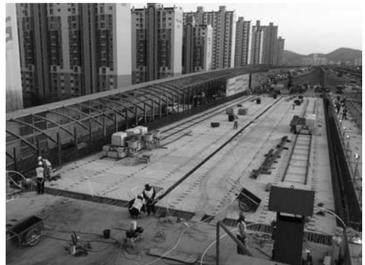
Figure 1. Replacement of fire-damaged bridge.
