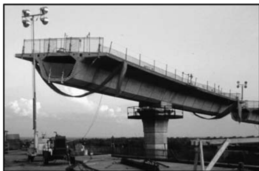
Figure 1. Balanced cantilever construction (I-35 inter-change, Austin, Texas).
