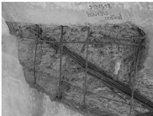
Figure 5. Brittle failure of wires of the KA prestressing kit.
