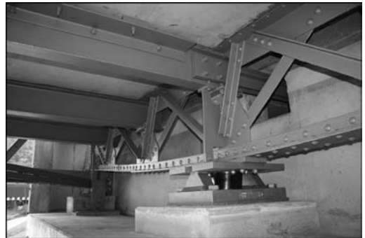
Figure 2. View of one abutment, showing bearing under central axis girder and tie-down anchorage of one edge girder. A new extension to the central axis girder passes through the abutment wall and connects to a new seismic damper.
