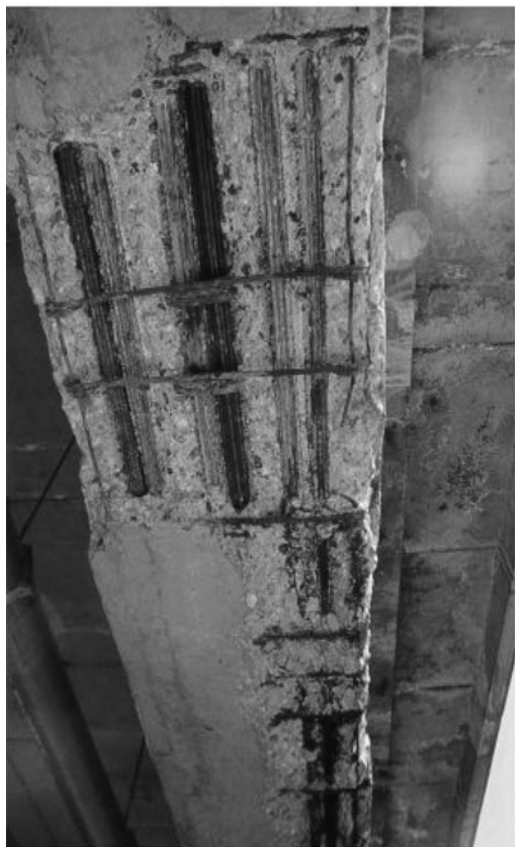
Figure 4. Illustration of the “random” distribution of corrosion.
