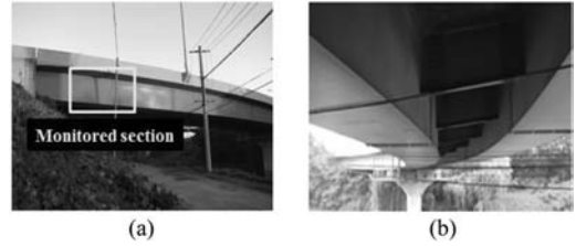
Figure 1. Overview of Ramp-G bridge in Goyang, Gyunggi, Korea: (a) Curved 90 m-long Ramp-G bridge and monitored section and (b) Two steel box girders.
