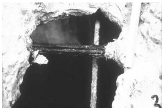
Figure 2. Condition of a transversal tendon located in the slab below the drainage channel.
