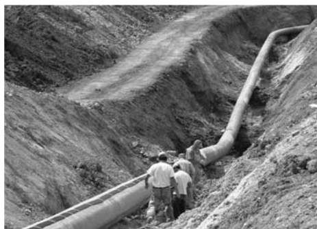
Figure 2. Pipeline strain monitoring in a landslide area in Italy.
