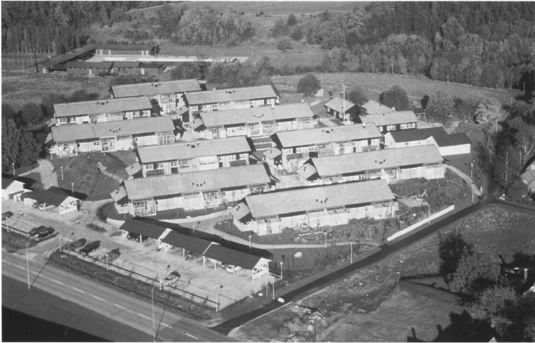
13.1 Low energy village at Lund, Sweden designed by Krister Wiberg (general view (top) and detail (bottom)).
