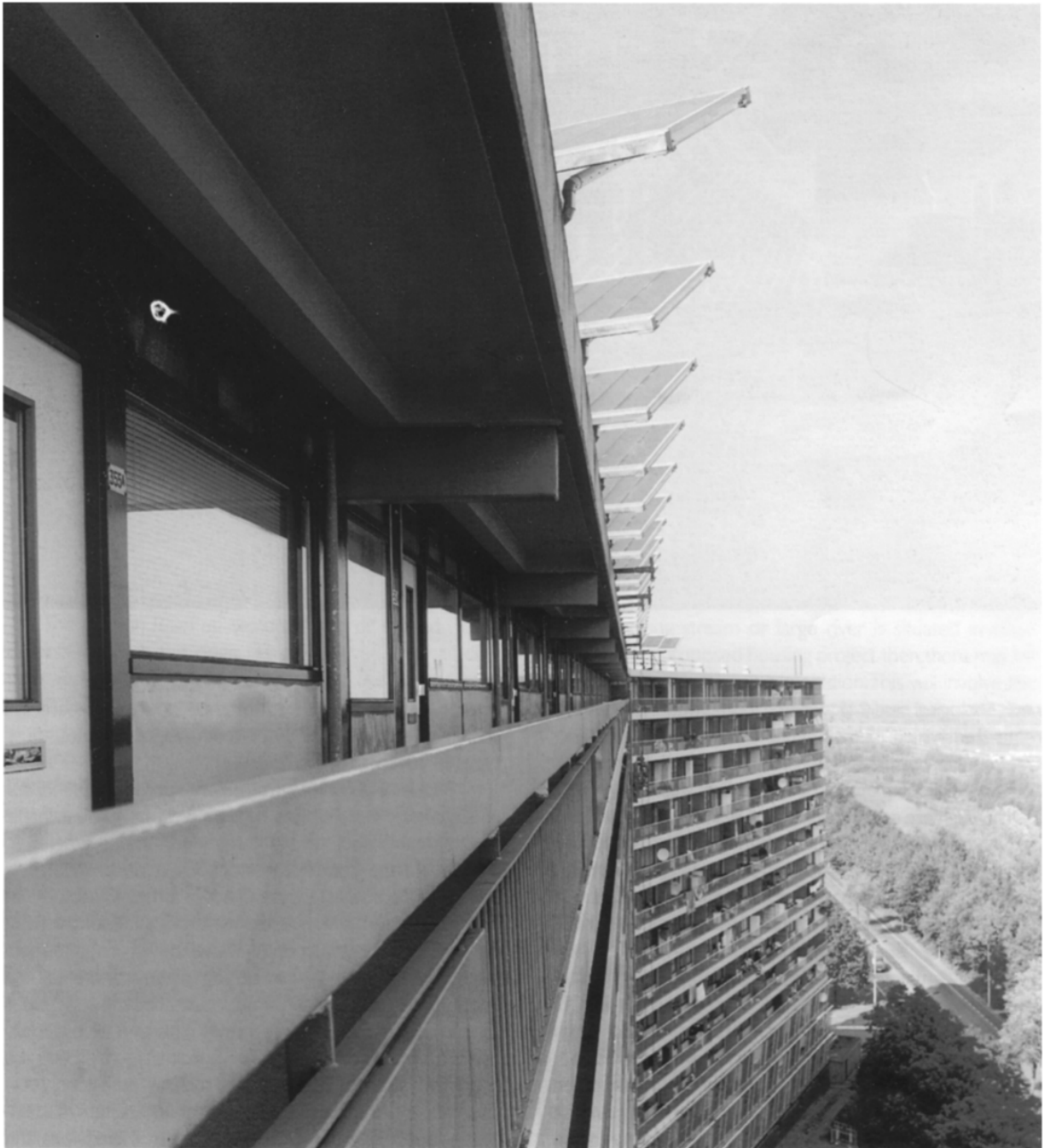
6.4 Solar thermal collectors used on the roof of an existing housing block in Zaandam as part of energy upgrading. Architect Hans van Heeswijk
