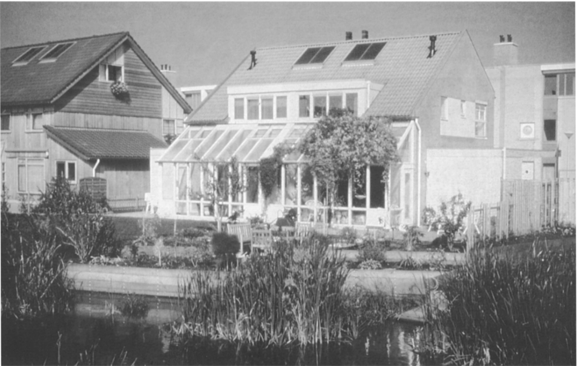
6.3 Houses in Ecolonia spread to the lakeshore which uses reedbeds to purify the greywater (opposite).
