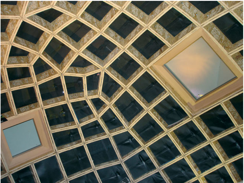
Fig. 5: Bottom-up-design: The CAAD/ETH Zurich Pavilion at the Swissbau-Messe 2005. The structure of the pavilion was optimized using artificial life methods. The structural mesh is shaped in a dynamic process by interaction between the individual hubs themselves and their surroundings (the openings and the spherical facade). The various nodes are shifted and added in accordance with certain regulations until specific structural specifications are fulfilled.
