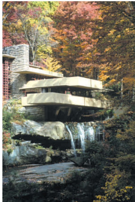
Frank Lloyd Wright's Fallingwater House in Bear Run, Pennsylvania
