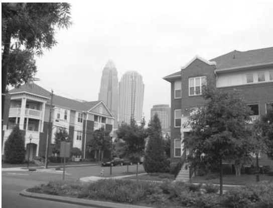
Figure 2.14 First Ward Place, Charlotte, NC, 1997–2001. Under the auspices of the US government's HOPE VI program, and following New Urbanist design principles, several cities have transformed blighted urban areas into attractive mixed-income neighborhoods like this Charlotte example.
