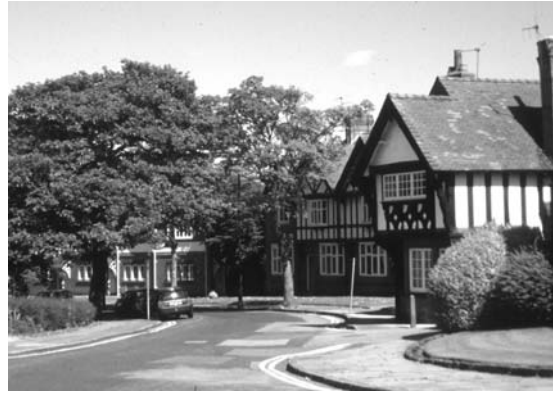
Figure 2.4 Port Sunlight, near Liverpool, UK, begun 1888. Soap magnate William Lever employed over thirty architects in the design of this industrial model village. It is characterized by picturesque groupings of traditional buildings in counterpoint to the long, neo-classical that forms the axis of the plan leading to the Lady Lever Art Gallery, completed in 1922.
