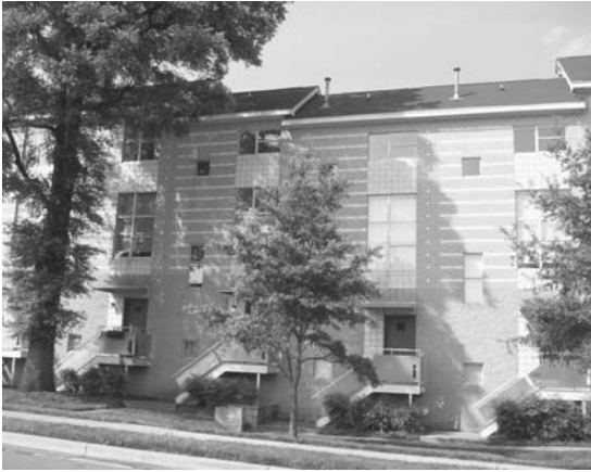
Figure 6.22 Atherton Heights, Dilworth, Charlotte, NC, David Furman, architect, 1998. This low cost housing organizes the proportions of its façade by tying together different sized openings with patterned brickwork on a predominantly solid wall.
