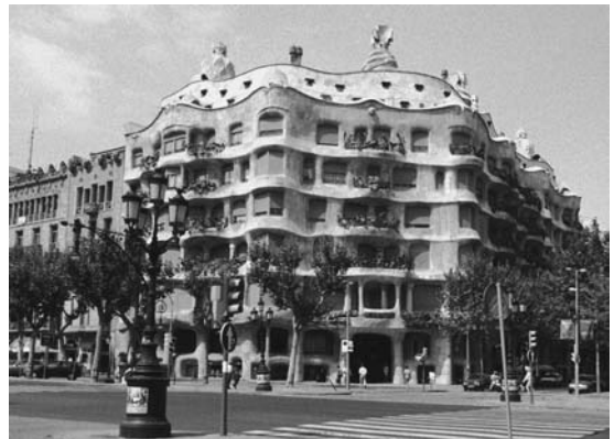
Figure 5.10 Casa Mila, Barcelona, Antonio Gaudi, 1906–10. Gaudi’s building obeys the dictates of Ildefonso Cerdá’s urban regulations with a simple plan that follows the required height and massing with its 45-degree corner splay. But within the apartments, Gaudi explores very sophisticated spatial rhythms, and his urban façade pulsates with idiosyncratic detail. Even greater freedom is evident on the roof, which is a riot of sculptural ornamentation. All this architectural invention occurs within a tightly controlled urban frame, and is all the more resonant because of this contrast.
