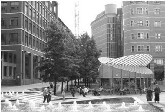
Figure 6.2 Central square, Brindleyplace, Birmingham, UK. Urban design master plan by John Chatwin, 1993. Decayed canalside land has been reclaimed as an exciting, productive mixture of uses through a comprehensive urban design master plan, good contemporary architecture and the careful design of the public spaces.
