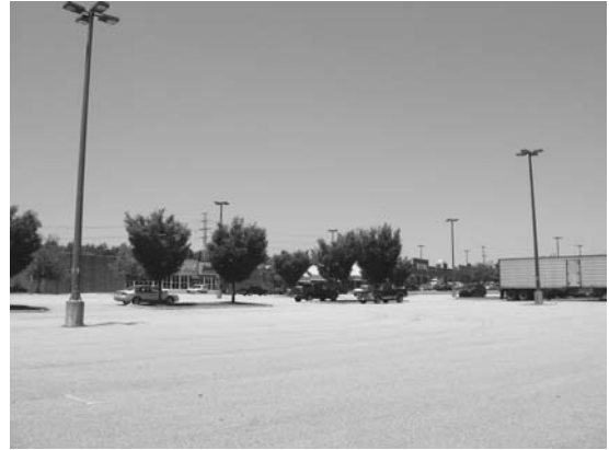
Figure 6.33 Parking lot, South Boulevard, Charlotte, NC. The standard American formula of large parking lots in front of stores created spaces for cars but nowhere that a normal human being could ever find hospitable. When the retail businesses fail, there is no other reason to be in these spaces, and the cycle of decline increases.
