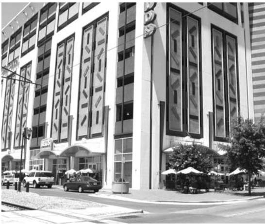
Figure 6.34 Seventh Street parking deck, Charlotte, NC. This parking deck, located on a new light rail line through the city center, features a grocery store and two restaurants on its lower floor. Its walls are enlivened by public art.
