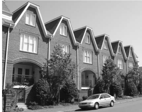
Figure 6.18 Townhouses, Mint Street, Charlotte, NC, 1998. The repetitive rooflines are dramatic, and bring a sense of appropriate scale to the row of houses without being fussy and over-ornamental.
