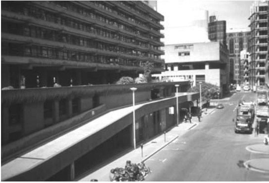
Figure 2.10 The Barbican, London, Chamberlain, Powell and Bon, 1954–75. This 40 acre (16 hectare) development in the heart of London extended the theme of separation of vehicles and pedestrians into the vertical plane. While this was a seductive urban theory, in practice the results were often inhuman. Streets were turned into dark service tunnels or canyons, while the pedestrian upper levels became little more than wind blown concrete wastelands. There is a pleasant urban space in the middle of the development around the Barbican Concert Hall, but this is small recompense for the brutal mutilation of the city fabric.
