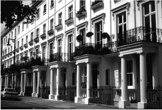
Figure 6.29 Nineteenth-century terrace in Belgravia, London. This view illustrates the power of repetition. Flat façades, so typical of nineteenth-century developers' architecture, reduce construction costs, but their potential boredom is relieved by the bold projection of entrance porches. Although identical, their vertical rhythms satisfy the eye and break the terrace down into identifiable units.
