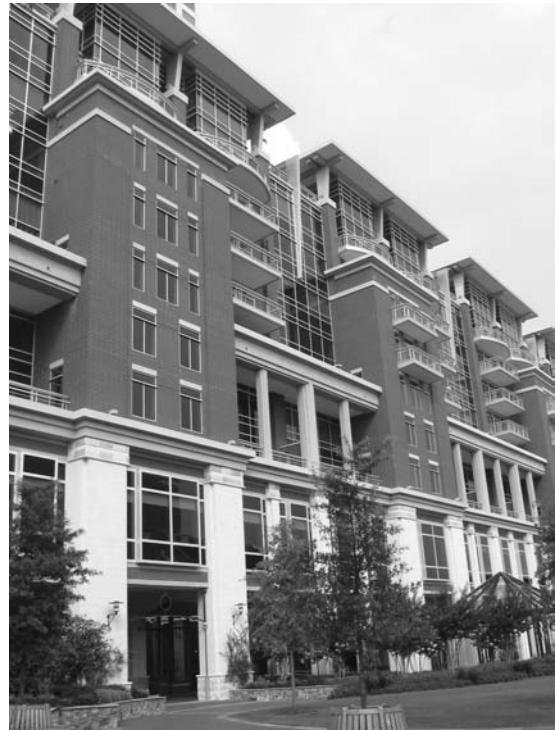
Figure 6.21 Radcliffe on the Green, Charlotte, NC, FMK architects, 2002. This block of luxury downtown housing above offices and restaurants creates complex rhythms and relationships to integrate a wide range of architectural elements across the façade.
