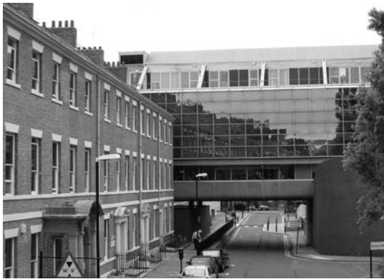
Figure 3.1 Office buildings, Newcastle-upon-Tyne, Ryder and Yates, architects, 1970. Many buildings from the 1970s were quite sophisticated structures. The office building on the left, for example, is designed as a giant beam from which the floors are suspended by cables enclosed in stainless steel cruciform mouldings, creating large open-plan floor areas. Despite such cleverness, buildings often demonstrated a crushing insensitivity to their context and the urban scale of the city. Other buildings of the late modernist period were for less clever. The example in the photograph on the right is just terrible. The new slab has no redeeming features whatsoever. It is a testament to the aesthetic power of the adjacent Victorian building that it even holds its own against this monstrous intrusion into the city fabric. Such design outrages are particularly poignant in Newcastle, which has a marvellous early Victorian urban structure and architectural legacy.
