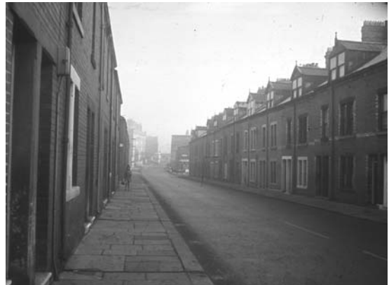
Figure 5.7 Street in Benwell, Newcastle-upon-Tyne, 1970. Typical workers' housing on the banks of the industrial River Tyne in northeast England used the 'Tyneside flats' – terraced houses divided into upstairs and downstairs apartments – to increase density. Front gardens and setbacks were non-existent, back yards were miniscule (just large enough to hold the outside lavatories and a short clothes line) and recreational spaces such as parks or playgrounds were never considered. Every piece of space was devoted to maximizing profit for the developer.
