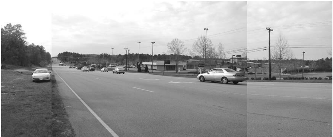
Figure 7.5 RTP Service Center, as existing. This photo-collage illustrates an undistinguished collection of buildings with no spatial cohesion or sense of place. Compare with Plate 20.
