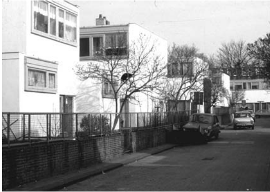
Figure 1.3 Kiefhoek Housing Estate, Rotterdam, J.J.P. Oud, 1925–29. Until Le Corbusier's doctrines were embodied in the all-encompassing Athens Charter of 1933, other modernists pioneers such as Oud were reluctant to abandon the street.
