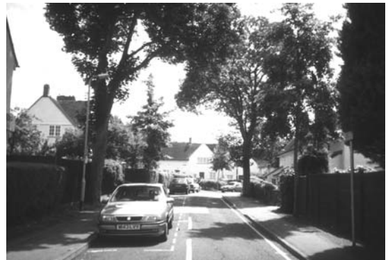
Figure 2.7 Housing at Letchworth Garden City, Parker and Unwin, 1904. Parker and Unwin progressively refined their techniques of housing design and layout. Note the attention to three-dimensional composition with a gable form terminating the visual axis while the street curves away to the right.
