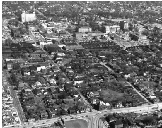
Figure 1.5 The Brooklyn neighborhood, Charlotte, NC, USA, early 1950s. Every building in this African-American community but one or two on the urban blocks in the fore and middle ground of this aerial view were demolished in the federally funded urban renewal programs of the 1960s. The area is now dominated by extensive complexes of government buildings, parking lots, and a large church with a white congregation. A new plan has recently been completed that will, over time, restore part of the block structure and promote mixed income housing. (Photo courtesy of the Charlotte Historic District Commission)
