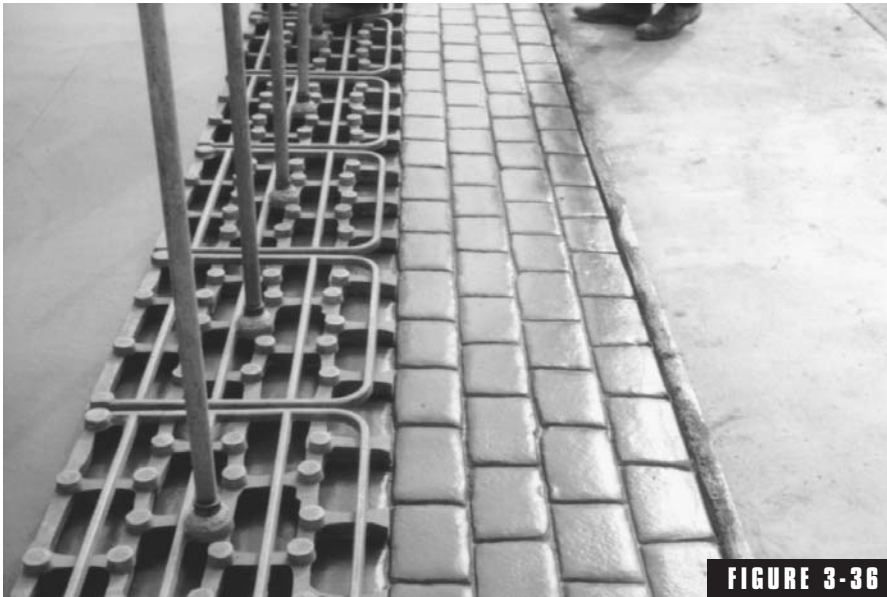
Pattern stamped concrete. (Photo courtesy PCA).
