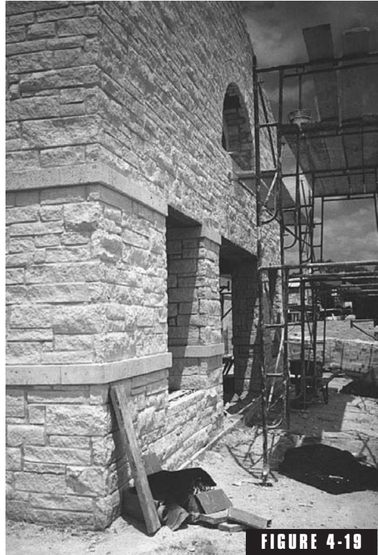
Rubble stone and ashlar used together.
