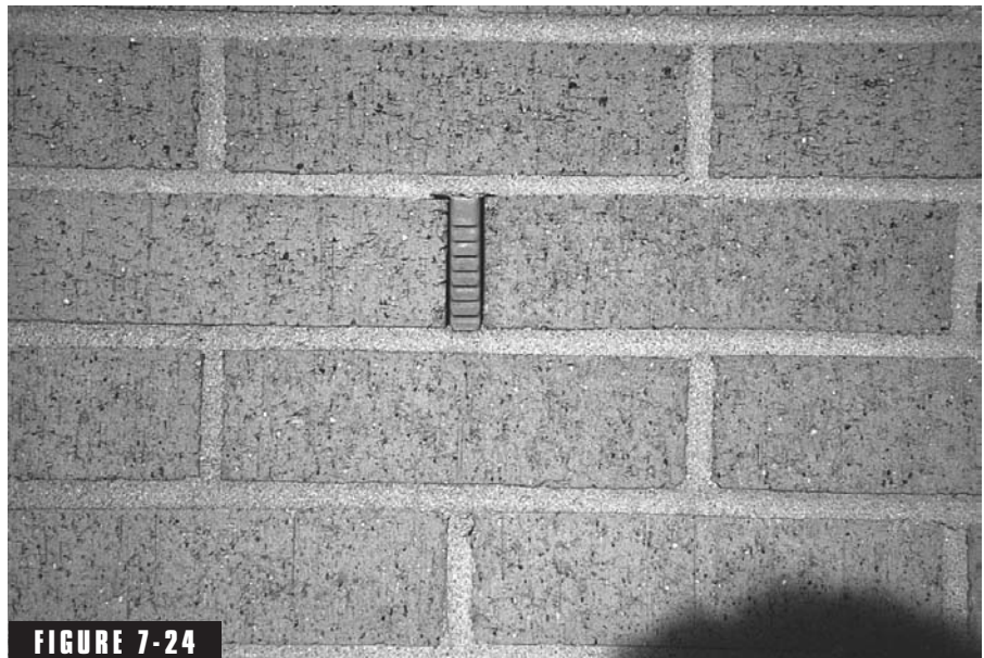
FIGURE 7-24 Weep hole vents.
