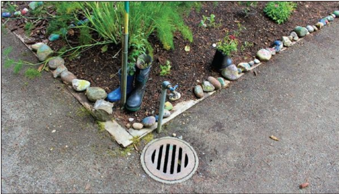
Zone 1 irrigation and controlled garden beds.
