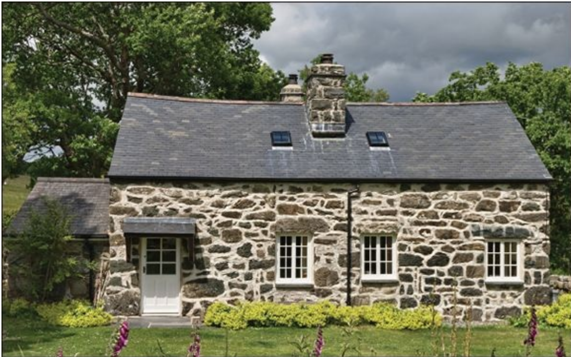
Slip form concrete house.
