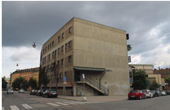
School of Architecture, The Royal Institute of Technology. One of the few Brutalist-style buildings in Stockholm. Above: The facade facing the city. Below: The same building seen from the partially fire-razed section. Photos: Carolina Krupinska
