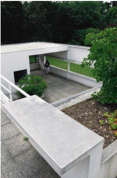
Villa Savoye, Poissy, France (completed in 1931) illustrates Le Corbusier's five rules for modern architecture: 1) the house on pilotis, 2) the free facade, 3) the open floor plan, 4) ribbon windows, and 5) a roof garden. Photo: Christian Ahlskog
