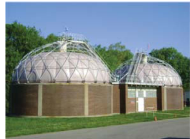
Figure 23.5 Anaerobic digestion operations—schematic and photo of standard single-phase digester.
