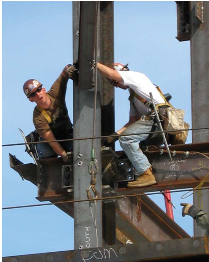
Figure 22.15 Constructing a steel frame. Worker safety continues to be one of the key performance measures of activities at the construction phase.
