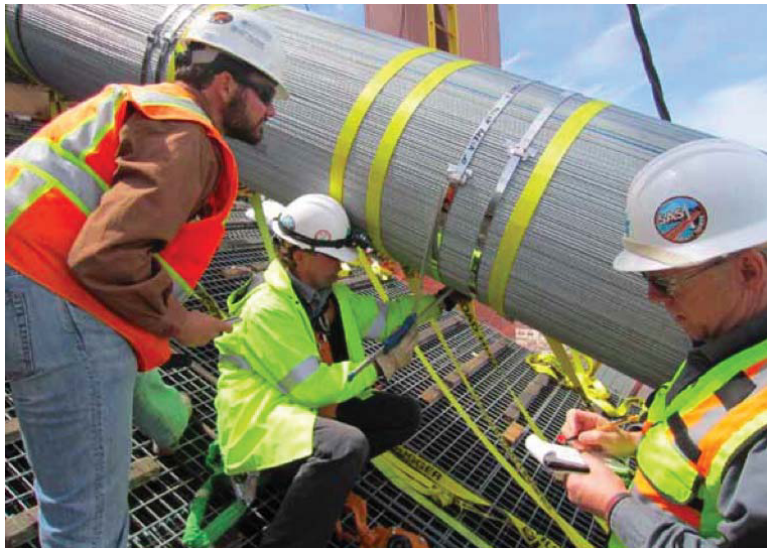
Figure 22.9 Inspectors test the adequacy of cable compaction during the reconstruction of the eastern span of the San Francisco–Oakland Bay Bridge [Courtesy of California Department of Transportation (Caltrans)].
