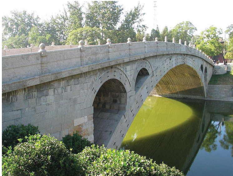
Figure 3.8 The Zhaozhou Bridge, China's oldest standing bridge and the world's oldest open-spandrel arch bridge, combines functionality and aesthetics (Courtesy of Zhao1974/Wikimedia Commons).
