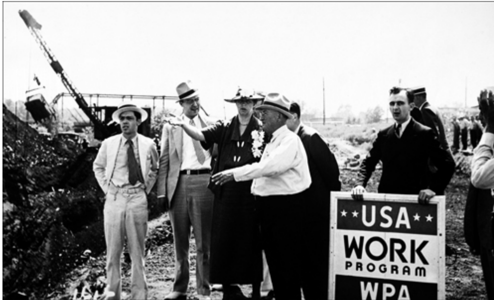
First Lady Eleanor Roosevelt visits a construction site of the Works Progress Administration in 1936. The central New Deal program to combat joblessness, the WPA provided jobs to some 8.5 million Americans—many on public works projects—over eight years. (The Granger Collection, New York)
