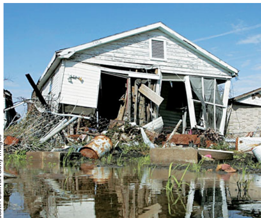
Was the Damage from Wind or Water? During Hurricane Katrina in 2005, high winds were confounded with high water so that often it was not possible to determine whether property damage was due to wind (insured) or to water (not insured).
