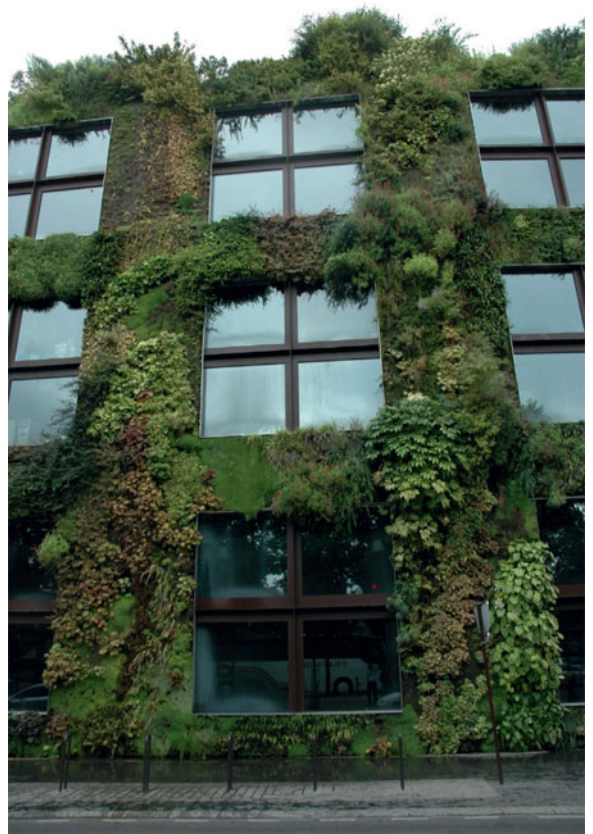
A “living wall” or “green wall” is a wall that is completely or partially covered with plants, as shown here at the Musée du Quai Branly in Paris.
