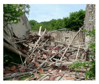
**Figure 20.5.** Suddenly collapsed barn, due to unknown adequate cause. During the past two hundred years, the barn suffered from bad maintenance. (Source: http://www.grenois.com/buurschuur.)
