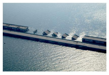
**Figure 21.1.** New Orleans, September 20, 2005. Sections of the eastern span of a causeway slid off their moorings and into the lake due to the winds and waters of Hurricane Katrina. (Photo: Win Henderson, Federal Emergency Management Agency (FEMA).)
