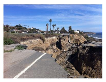
**Figure 20.1.** Landslide near San Pedro, California, on November 21, 2011. Rain exacerbated a slow-moving landslide that left large crevices on a road along the coast. The road broke into pieces that crumbled into gaping holes, while other sections fell into the ocean below. (Photo: USGS: US Geological Survey, www.gallery.usgs.gov/afv2YLk885/large/san\_pedro\_landslide\_knabe.jpg.)
