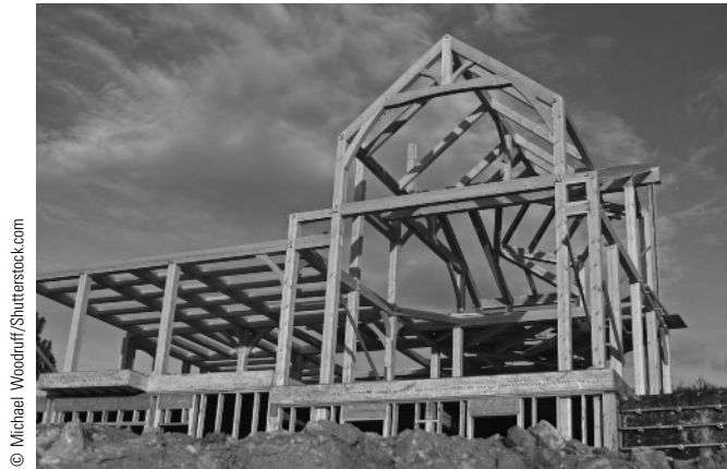
Framing a house is a major deliverable in a house project.
