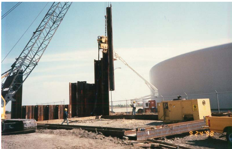
FIGURE 7.5 Pile driving operation using vibratory hammer.
