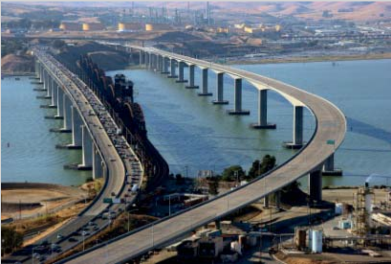
FIGURE 8.CS2 Benicia–Martinez Bridge completed looking from Martinez, California (courtesy of Kiewit Infrastructure West).
