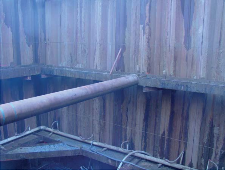
FIGURE 7.4 Sheet pile, waler, and strut system.
