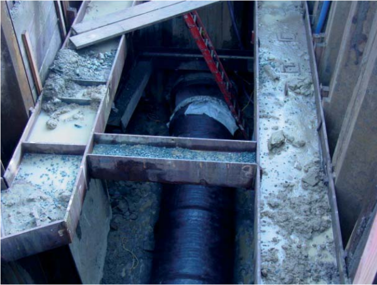
FIGURE 7.17 Strut supporting walers.
