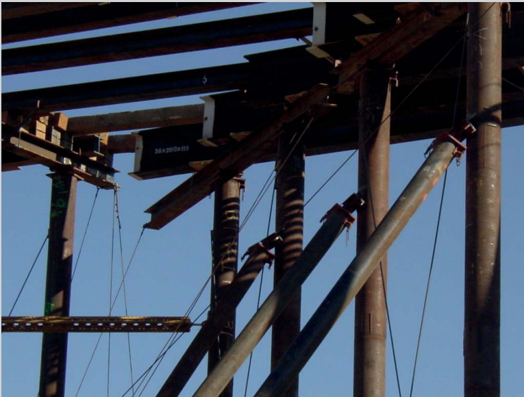
FIGURE 10.CS2 Push-pull braces added to falsework.
