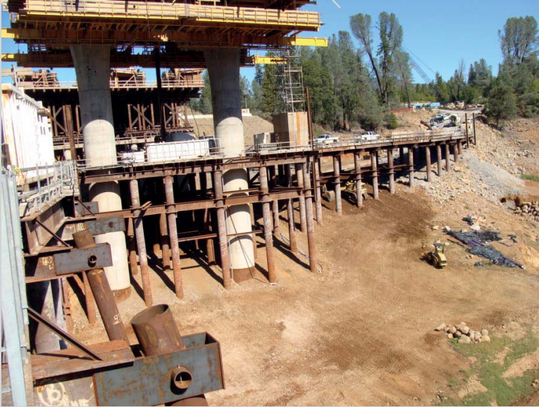
FIGURE 12.CS1 Trestle on north side of lake.
