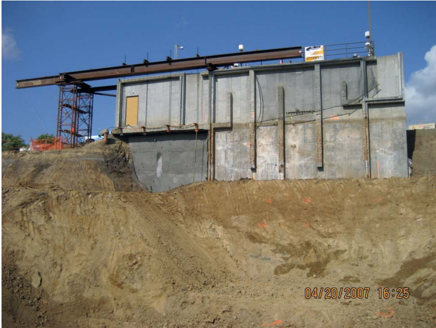
FIGURE 3.18 Temporary support of an existing structure.
