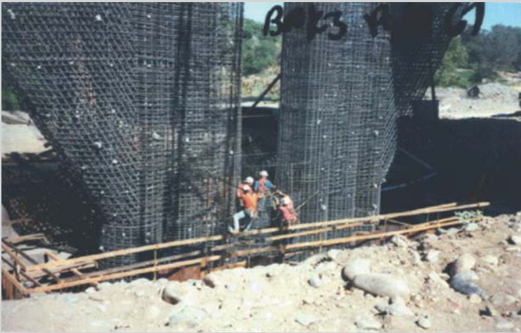
FIGURE 11.CS2 Installing braces.
