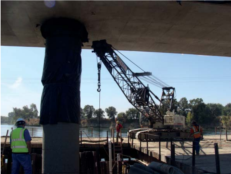
FIGURE 12.1 Driving sheet pile from work trestle.
