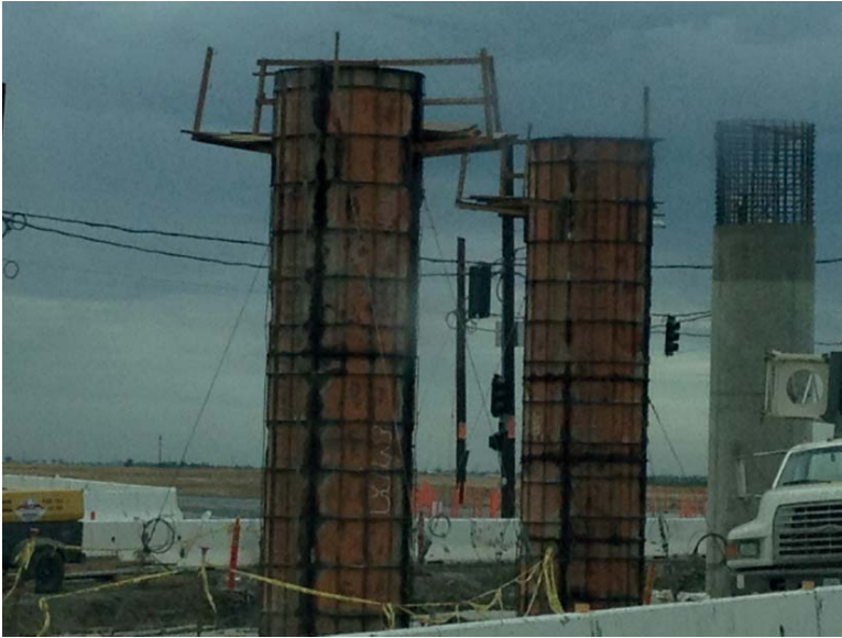
FIGURE 11.11 Pier forms guyed with wire rope.
