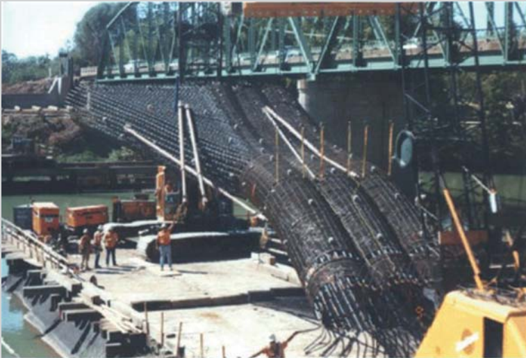
FIGURE 11.CS1 Hoisting of rebar cage.
