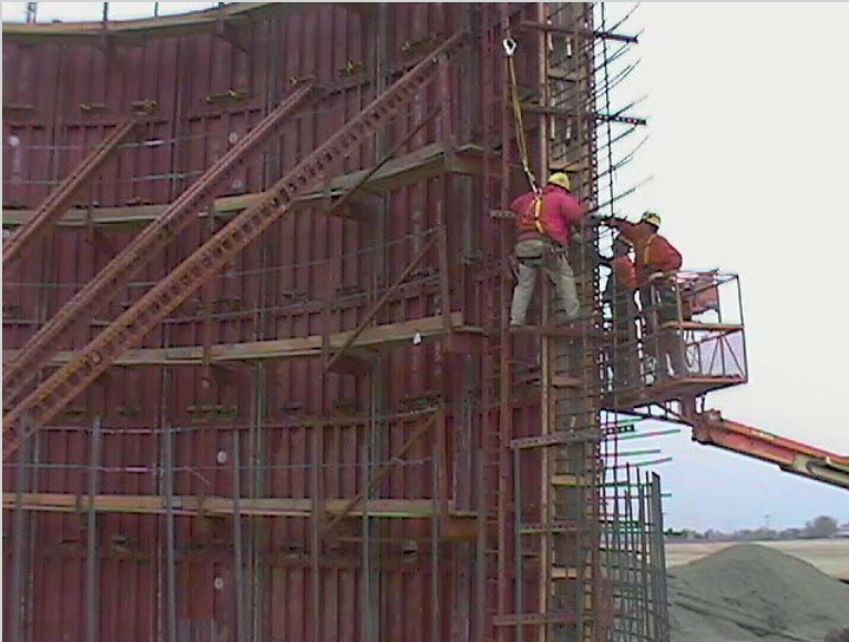
FIGURE 9.CS1 Steel forms used for a digester tank.
