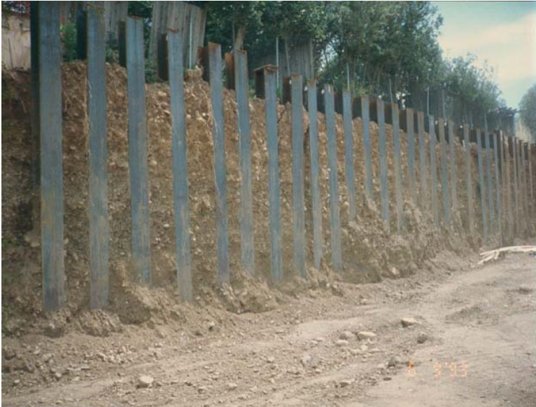
FIGURE 6.19 Soldier beams without lagging.
