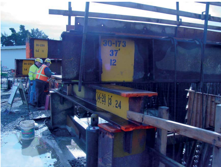
FIGURE 12.3 Stringer supported by cap beam.
