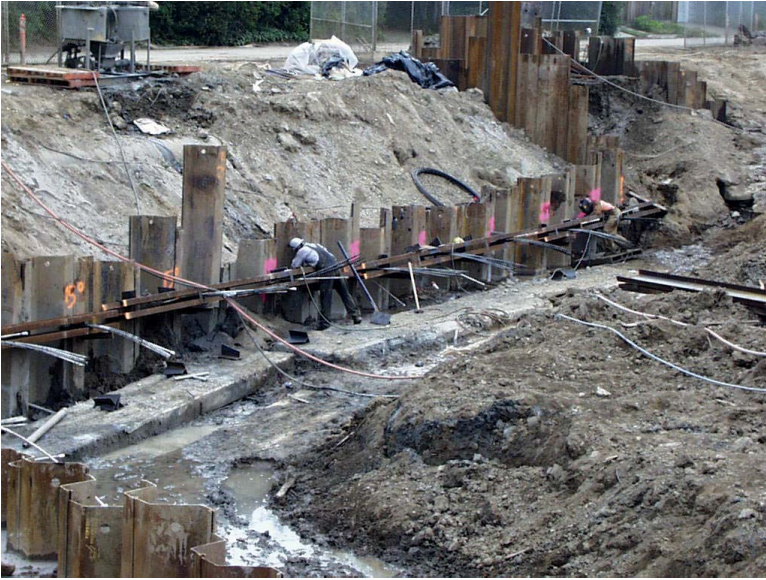
FIGURE 7.10 Double channel water system with tiebacks.
