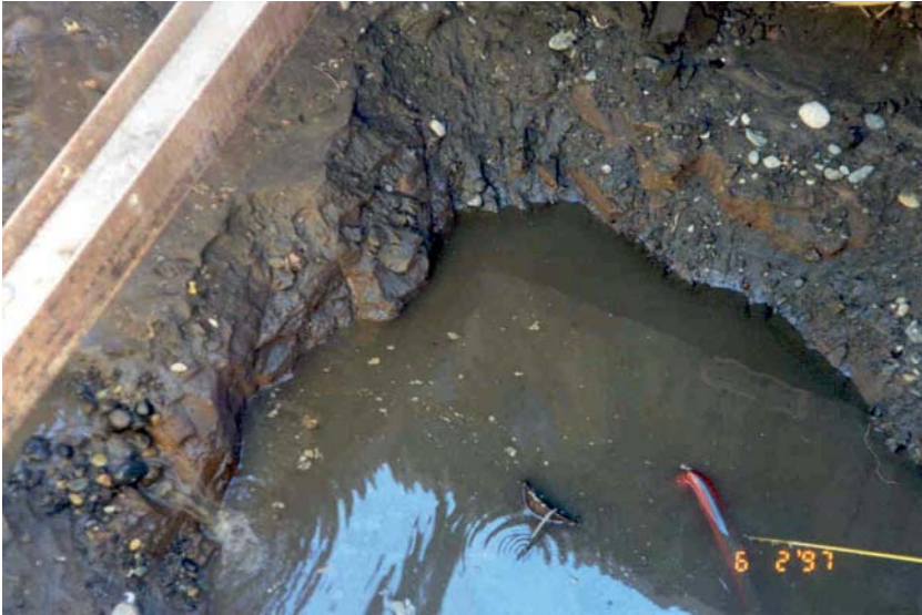
FIGURE 5.26 Soil conditions in a sheet pile cofferdam.
