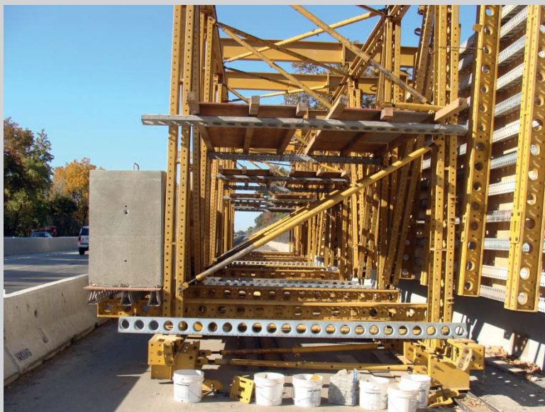
FIGURE 9.CS6 Traveling truss with counterweights.
