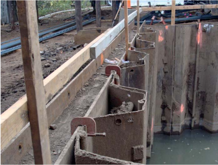
FIGURE 7.15 External waler system using bridge style C clamps.
