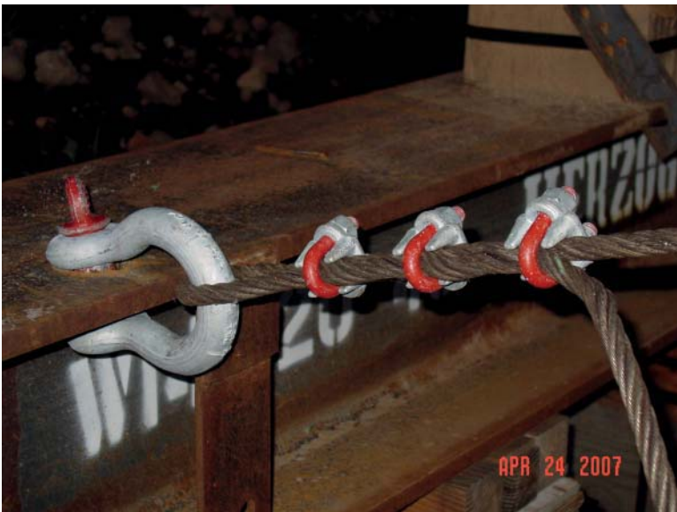
FIGURE 11.18 Wire rope connection with clips and thimbles.
