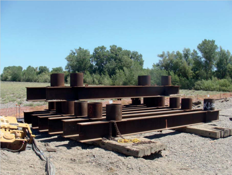
FIGURE 12.CS7 Prefabricated pile caps.
