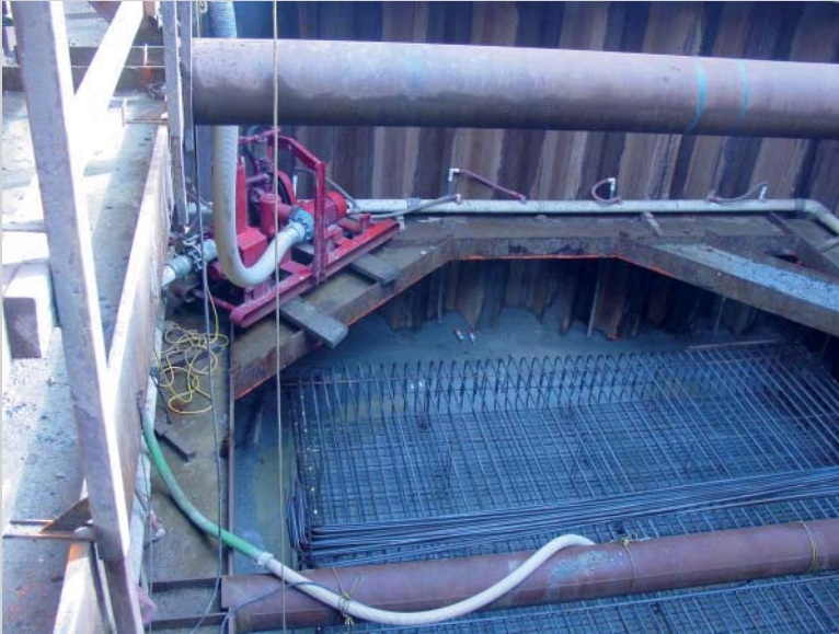
FIGURE 7.CS3 Sheet pile cofferdam (courtesy of Kiewit Infrastructure West).
