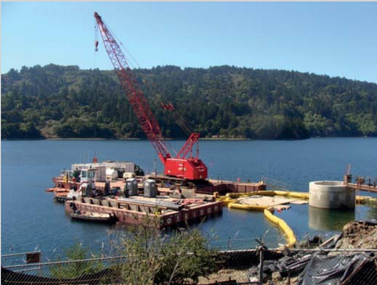
FIGURE 8.CS4 Barge arrangement for underwater work. (courtesy of Kiewit Infrastructure West)
