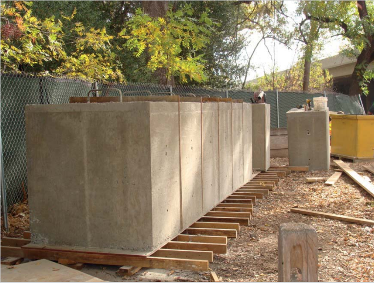
FIGURE 9.CS7 Counterweights (deadmen) on casting bed.
