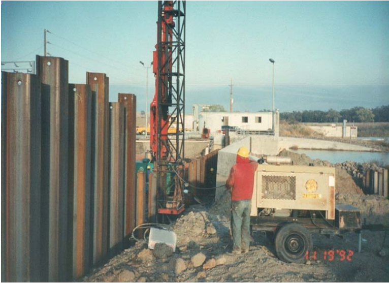
FIGURE 7.6 Sheet pile driving with an impact hammer.
