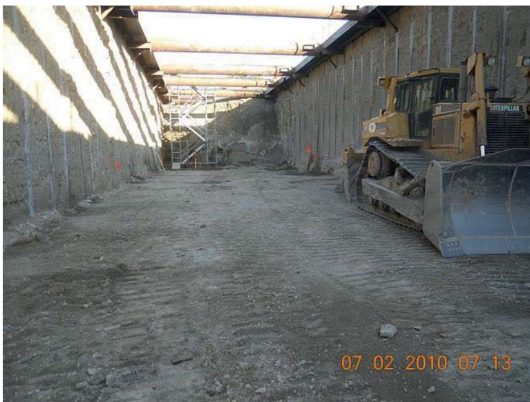
FIGURE 6.27 Deep soil mixing with soldier beams, Owner, Valley Transit Authority (VTA).
