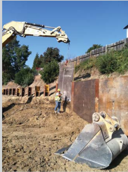
FIGURE 6.CS2 Plate installation.
