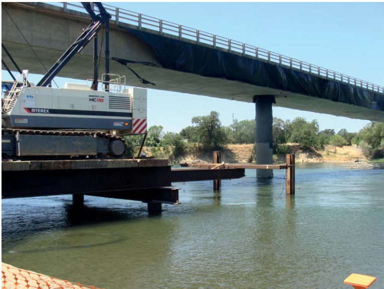
FIGURE 12.7 Work trestle over the Sacramento River.
