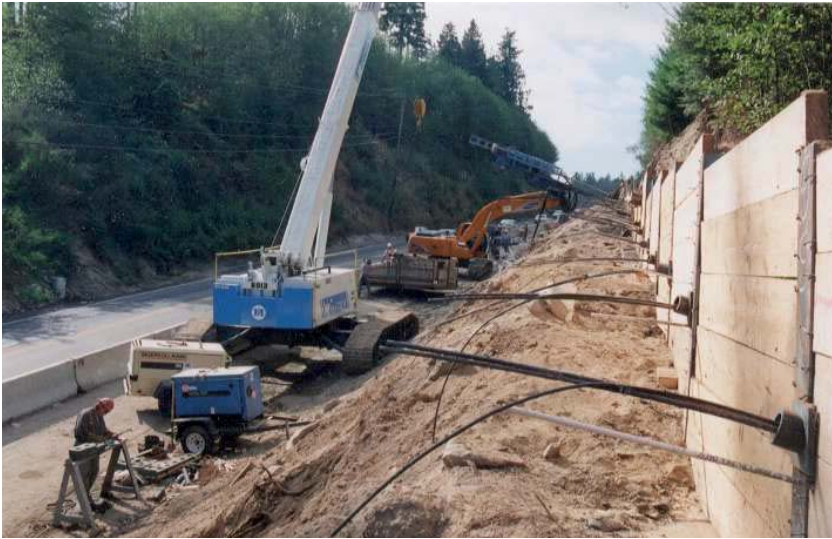
FIGURE 6.23 Soldier beam shoring with tiebacks.
