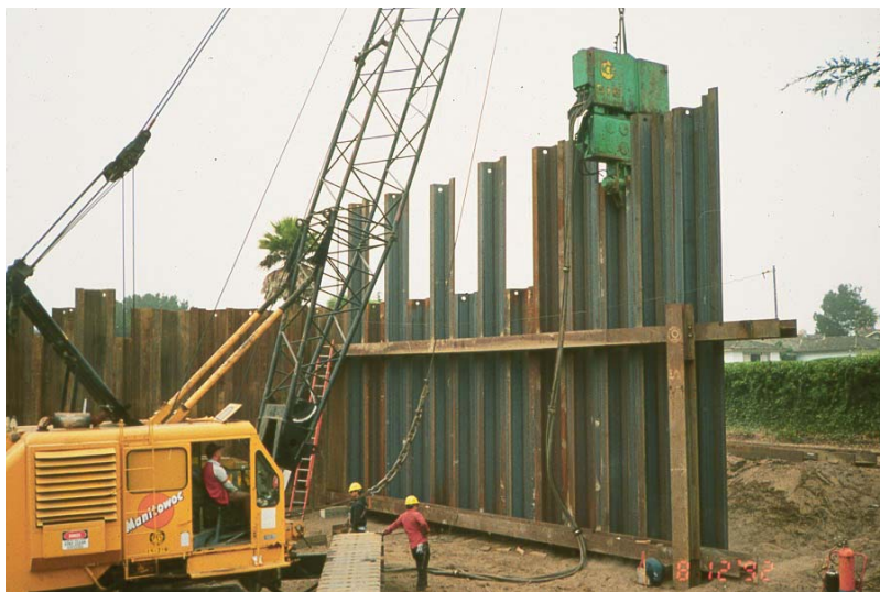
FIGURE 7.7 Two-tier driving template.
