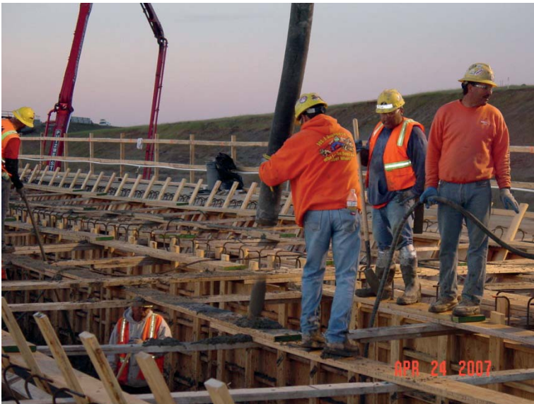
FIGURE 3.10 Concrete placement on a bridge superstructure.
