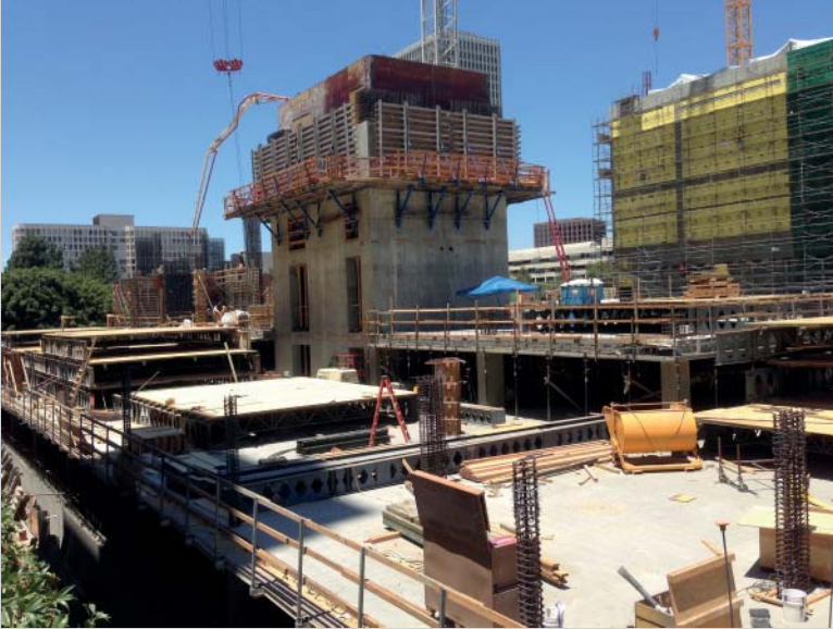
FIGURE 10.CS7 Jump form system (courtesy of Charles Pankow, Ltd and Doka Forms).
