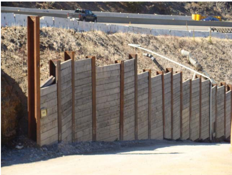
FIGURE 6.4 Cantilevered soldier beam system.
