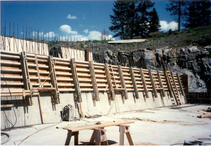
FIGURE 8.5 Monolith dam construction cantilevered form.
