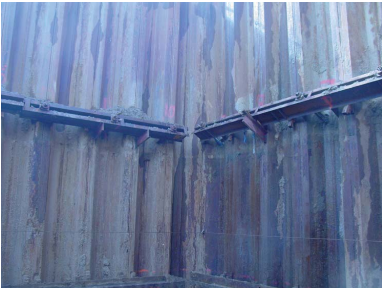
FIGURE 5.19 Double steel channel waler with tiebacks.
