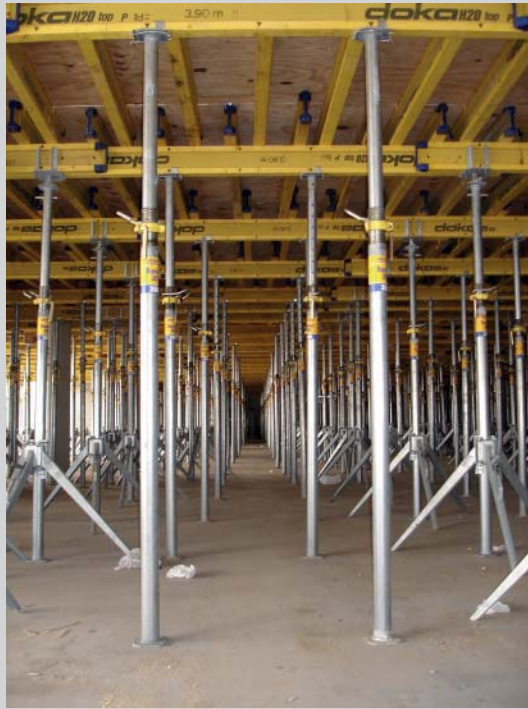
FIGURE 10.CS11 Doka form system (courtesy of Charles Pankow, Ltd and Doka Forms).
