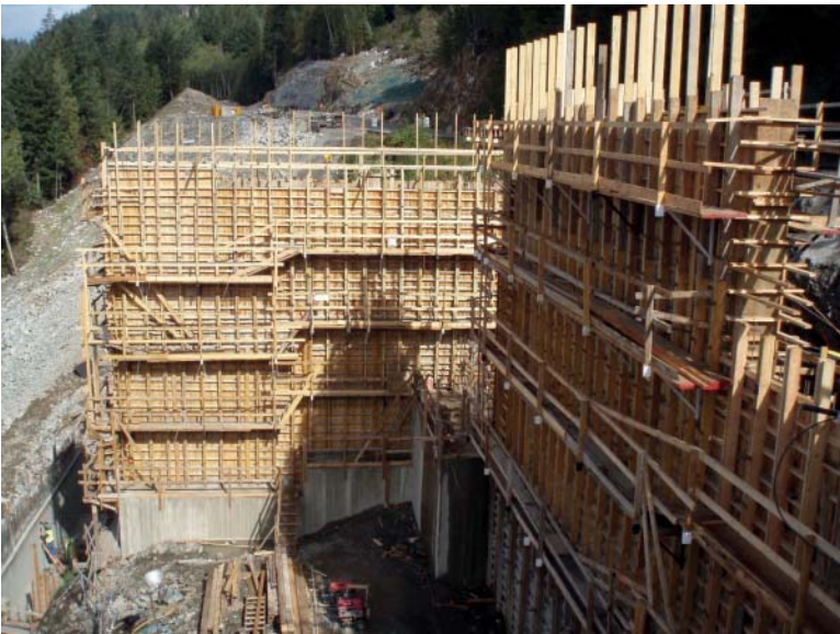
FIGURE 9.4 Typical 2 \times 4 and plywood formwork.
