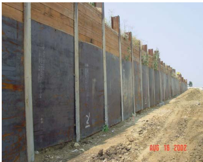
FIGURE 6.8 Combined wood and steel plate lagging.
