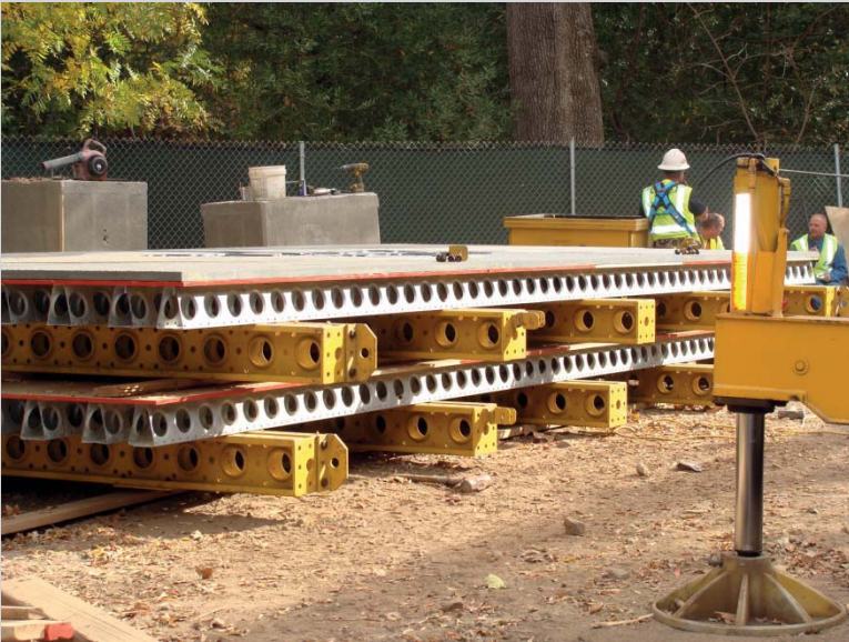
FIGURE 9.CS8 Prefabricated wall forms with form liner.
