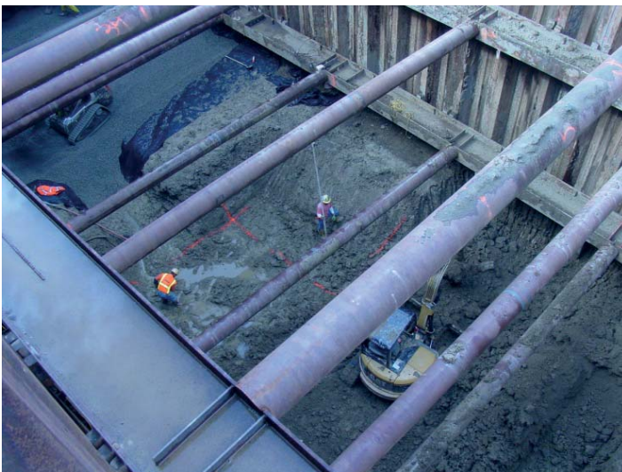
FIGURE 5.21 Multilevel supported excavation.
