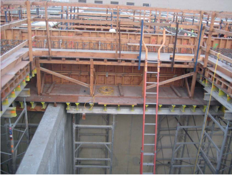
FIGURE 10.10 Slab and dropped beam.
