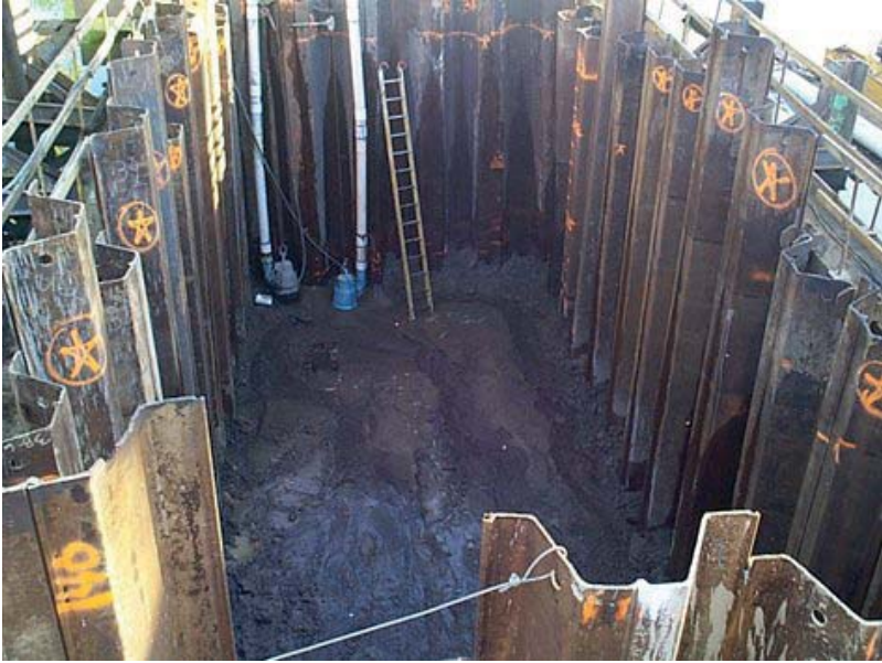
FIGURE 5.28 Sheet pile cofferdam with external walers.
