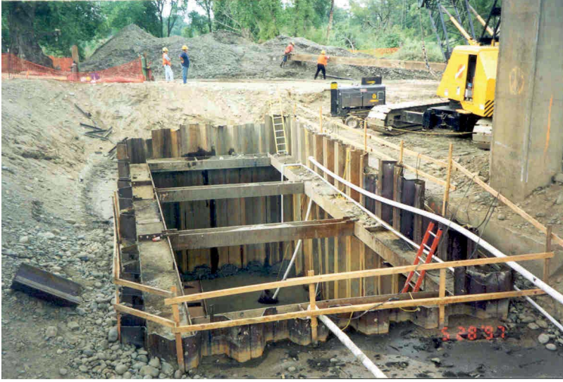
FIGURE 7.19 Struts used in a floodplain cofferdam.
