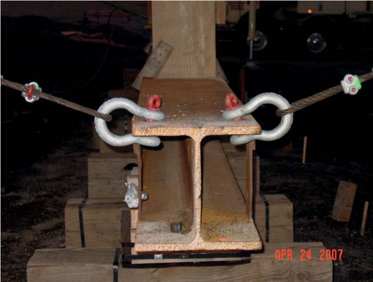
FIGURE 11.28 Longitudinal bracing connected to bottom cap.
