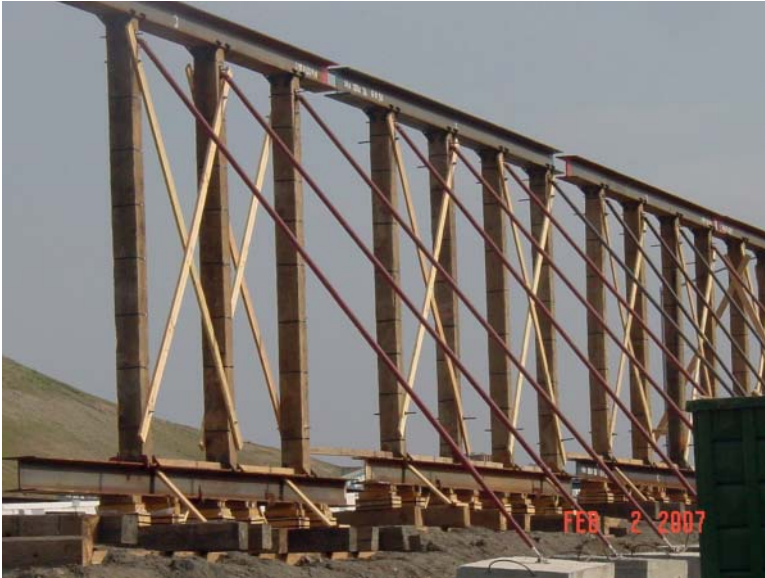
FIGURE 11.9 Falsework bent supported by pipe braces.
