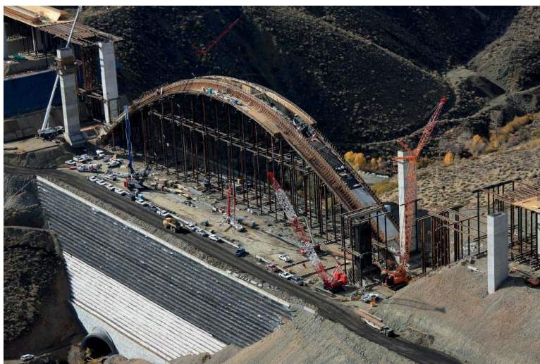
FIGURE 12.38 Galena Creek bridge.
