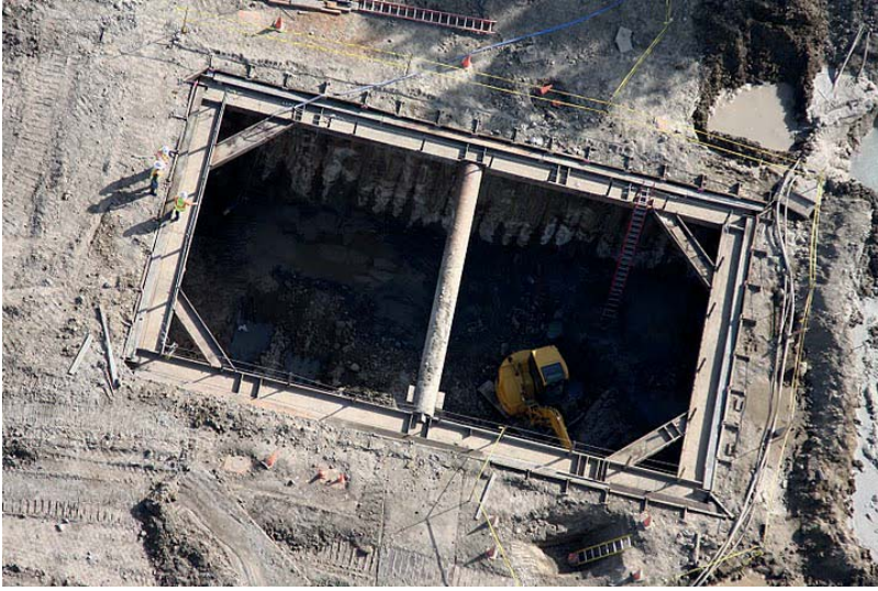
FIGURE 7.20 Aerial view of a struted cofferdam.
