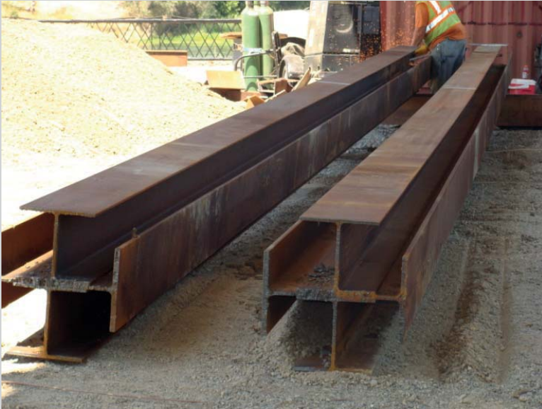
FIGURE 12.CS5 Star pile.
