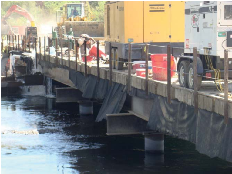
FIGURE 12.12 Trestle with wood decking.
