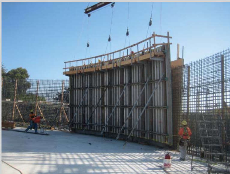
FIGURE 9.CS2 Aluminum and rolled steel channel radius forms.
