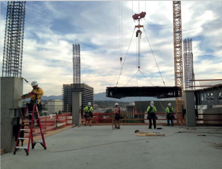
FIGURE 10.CS5 Fly table (courtesy of Charles Pankow, Ltd and Doka Forms).
