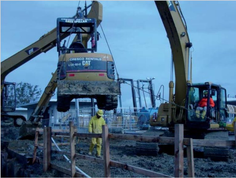
FIGURE 7.CS1 Sheet pile cofferdam (courtesy of Kiewit Infrastructure West).
