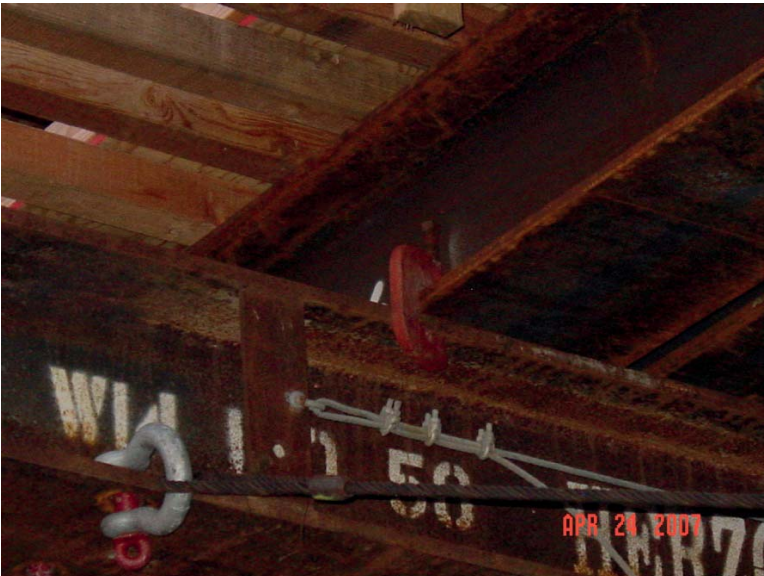
FIGURE 11.29 Beam clamp attaching a stringer to a top cap.
