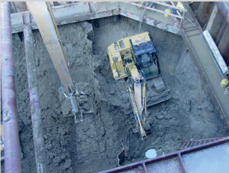
FIGURE 7.CS2 Sheet pile cofferdam (courtesy of Kiewit Infrastructure West).
