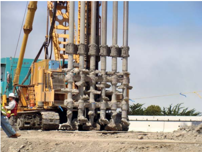
FIGURE 6.25 Deep soil mixing equipment Presidio Project, San Francisco.
