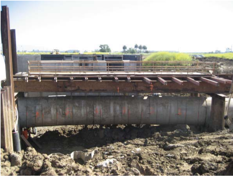
FIGURE 13.15 Pipe support.
