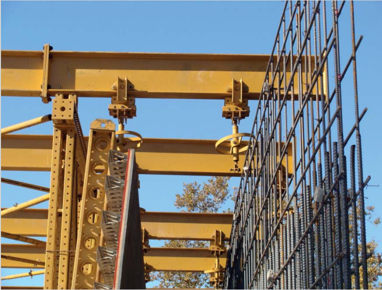
FIGURE 9.CS5A Inside and outside forms supported by cantilevered beam.
