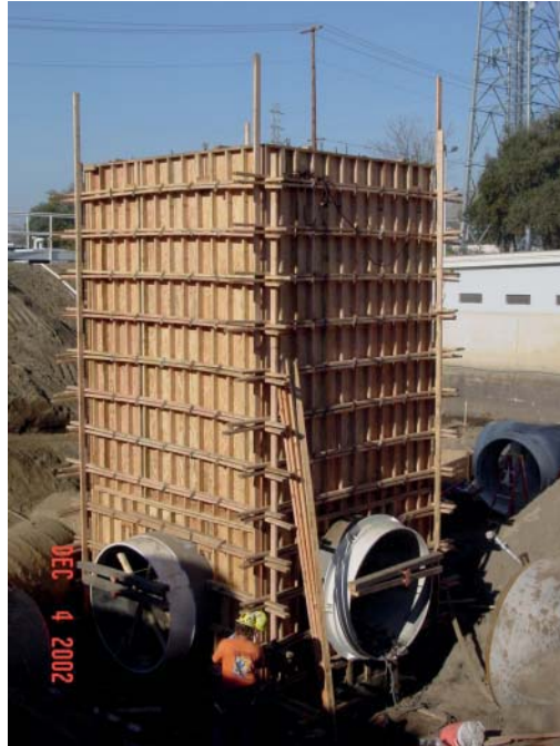
FIGURE 9.6 Junction box formed with all-wood forms.
