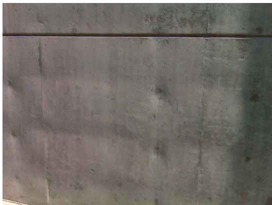
FIGURE 9.2 Plywood and stud deflection.
