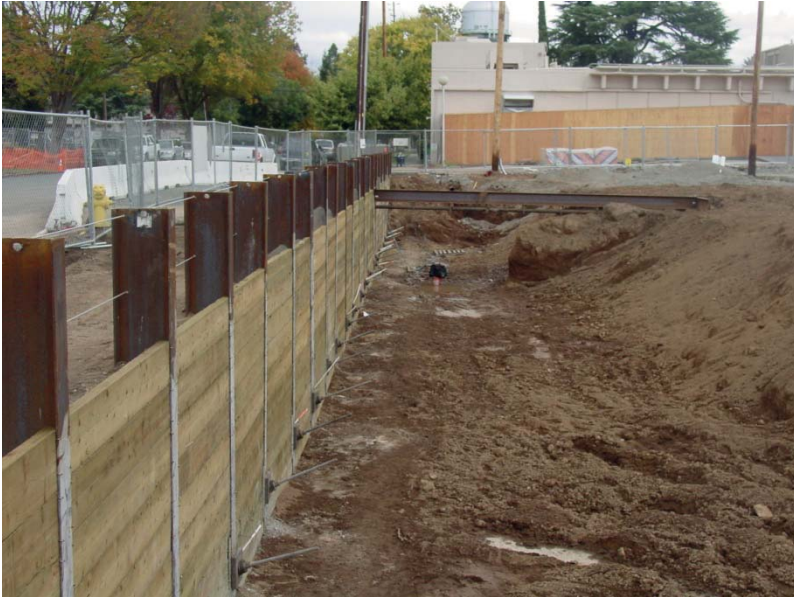
FIGURE 3.15 Soldier beam and lagging system.
