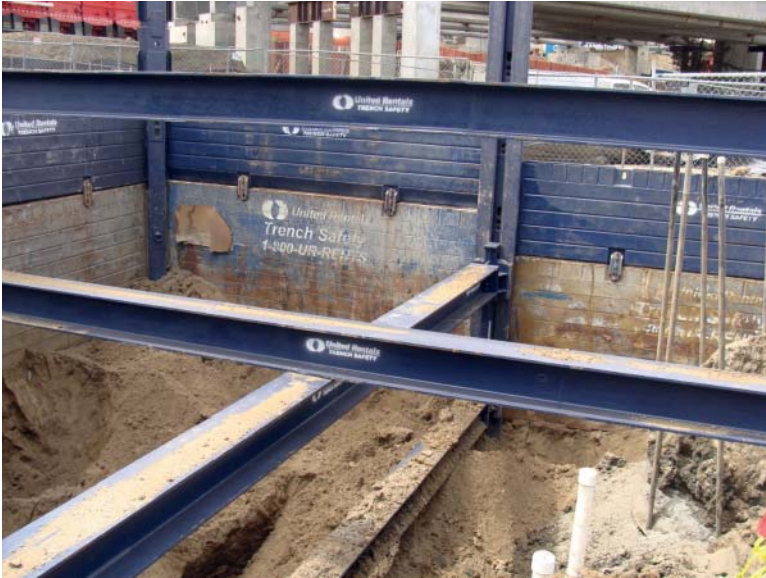
FIGURE 5.29 Slide rail system.
