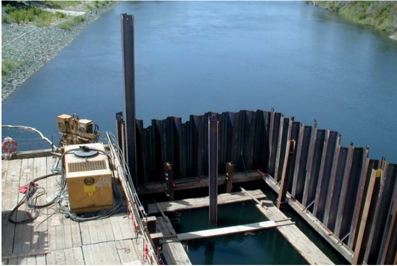
FIGURE 7.14 Internal waler in a river cofferdam.
