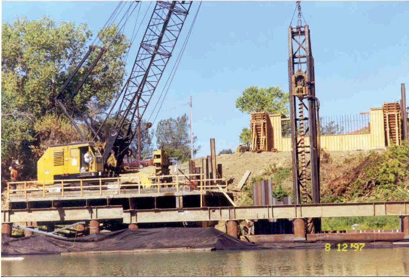
FIGURE 7.8 Predrilling a sheet pile line in the Feather River.
