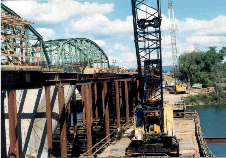
FIGURE 10.1 Pipe post falsework.
