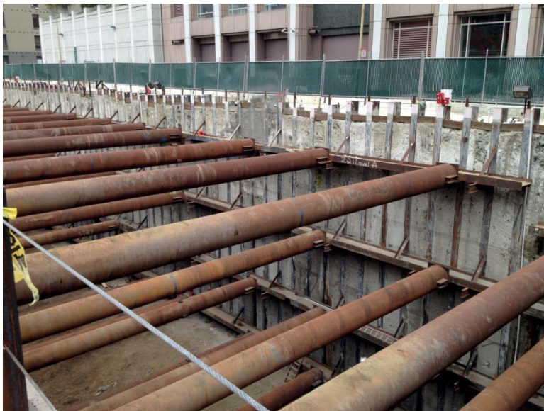
FIGURE 6.26 Multilevel walers and struts supporting soldier beam and deep-soil mix wall.
