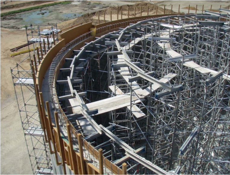
FIGURE 10.2 Water tank falsework using aluminum system.
