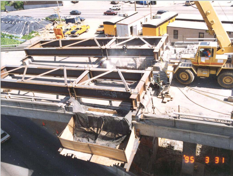
FIGURE 13.CS4 Hinge support.
