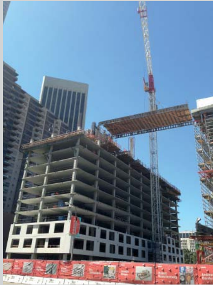
FIGURE 10.CS6 Fly table installation (courtesy of Charles Pankow, Ltd and Doka Forms).
