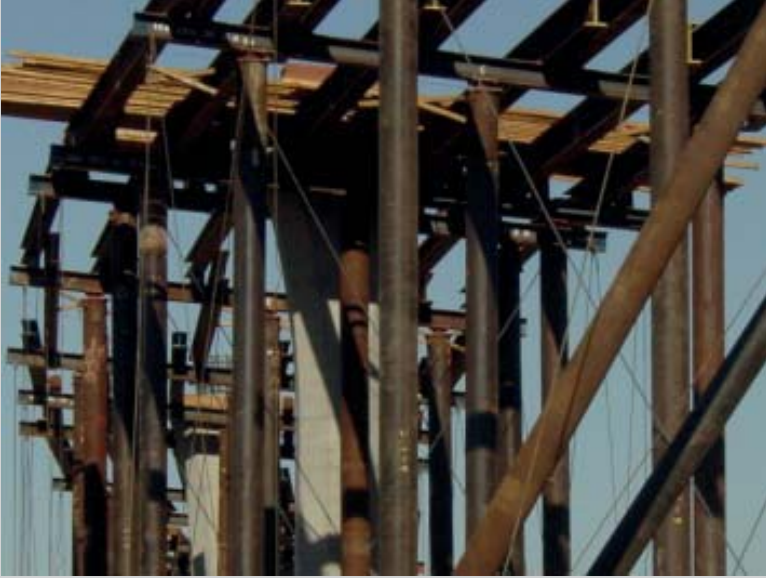
FIGURE 10.CS1 Typical falsework for this project.
