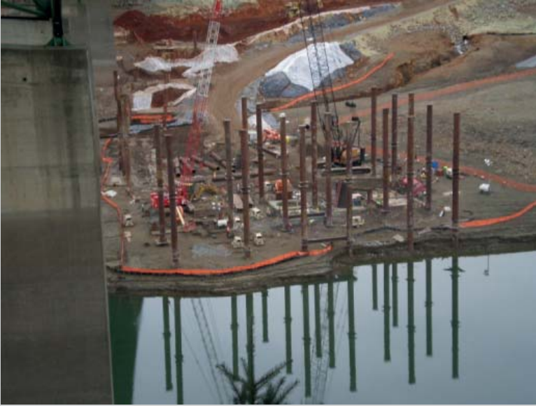
FIGURE 12.CS2 Trestle under construction—year 1.
