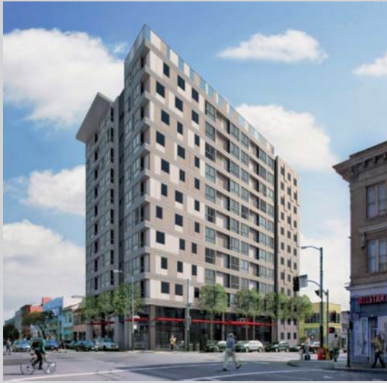
FIGURE 10.CS9 1321 Mission Street apartment building (Courtesy of Charles Pankow, Ltd and Doka Forms).
