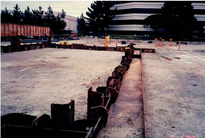
FIGURE 7.16 External waler using plate clamps.
