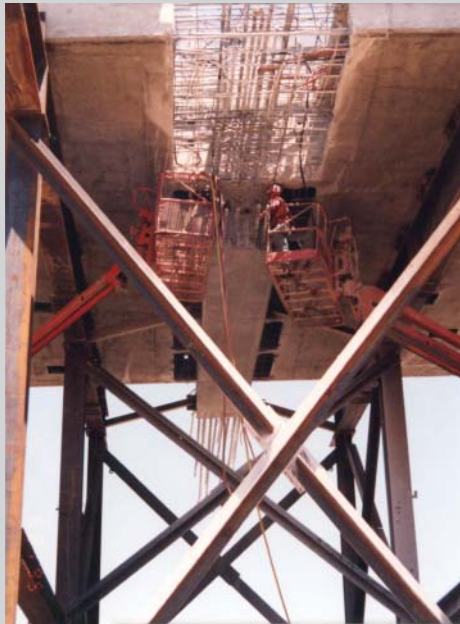
FIGURE 13.CS3 Typical bent cap replacement.
