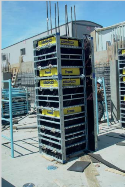
FIGURE 10.CS14 Column forms (courtesy of Charles Pankow, Ltd and Doka Forms).
