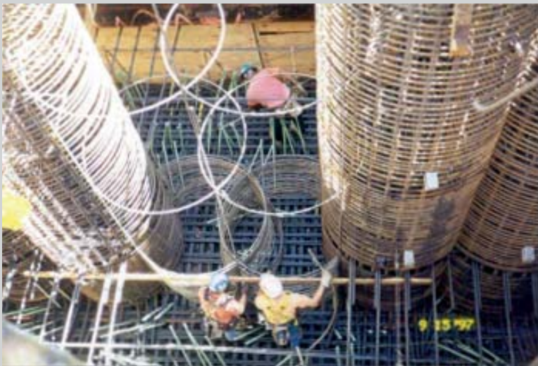
FIGURE 11.CS3 Placing of intermediate hoop reinforcing.
