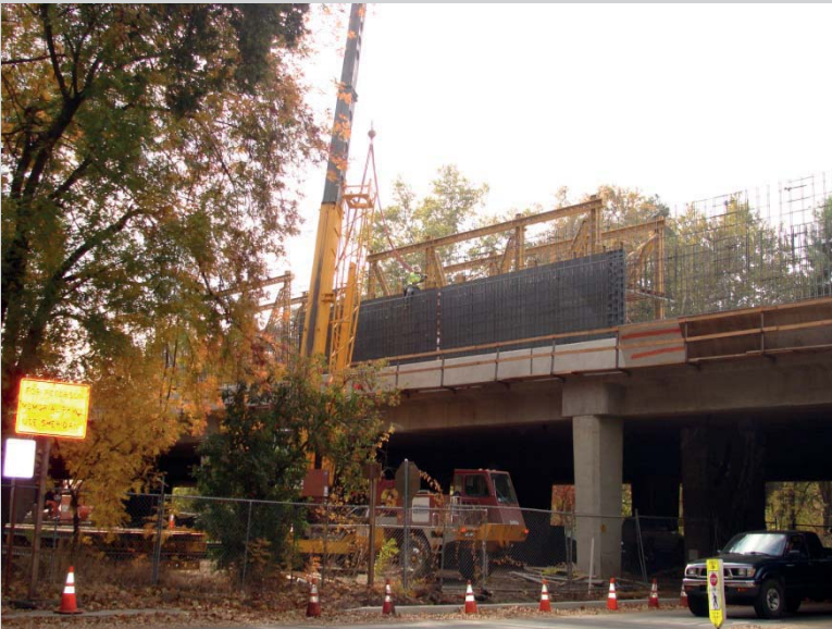
FIGURE 9.CS5B Crane hoisting first form into place.
