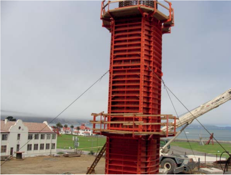
FIGURE 11.19 Pier guying system.
