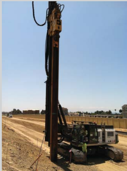
FIGURE 6.CS1 Soldier beam and plate system.
