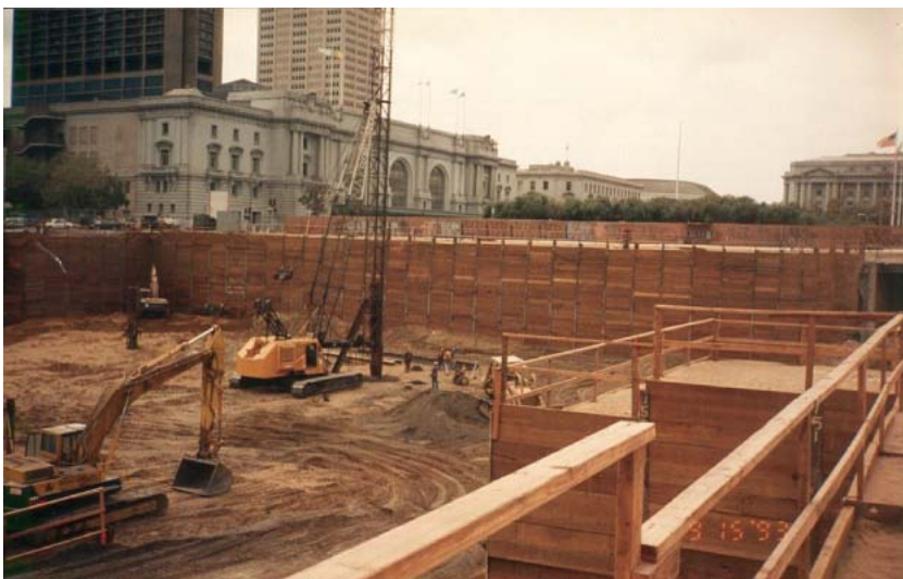
FIGURE 6.6 Lagging system in place.
