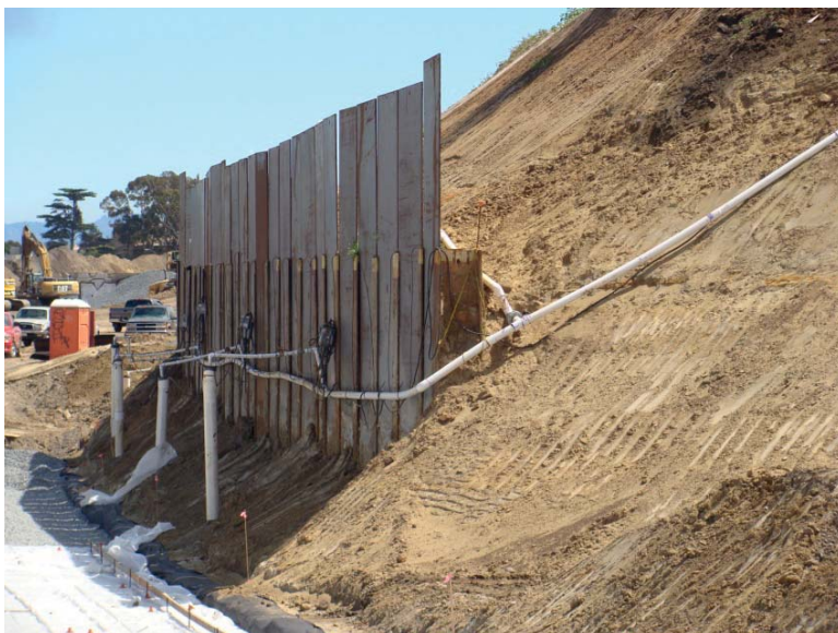
FIGURE 6.9 Soldier beam and plate with dewatering system.
