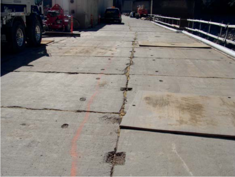
FIGURE 12.6 Precast concrete trestle deck.
