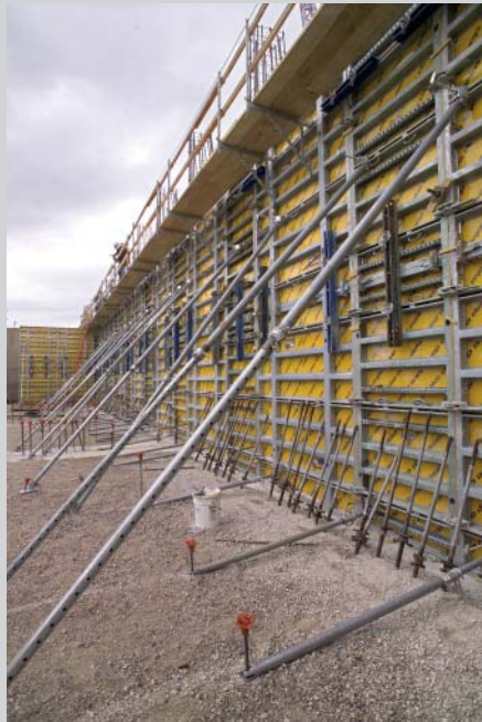
FIGURE 10.CS15 Wall forms (courtesy of Charles Pankow, Ltd and Doka Forms).
