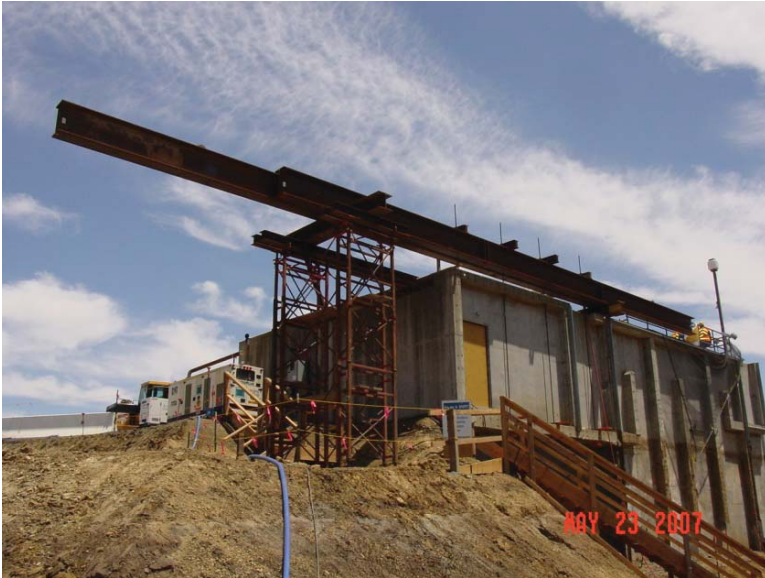
FIGURE 13.2 Temporary support of an existing structure.
