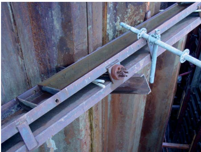
FIGURE 7.3 Double channel waler system before excavation.
