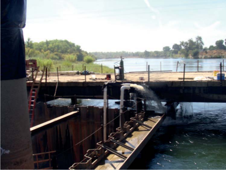
FIGURE 12.CS4 First season trestle—south side.
