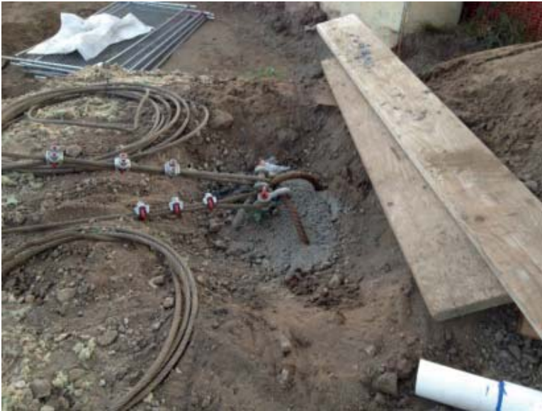
FIGURE 11.22 Drilled pile anchor.
