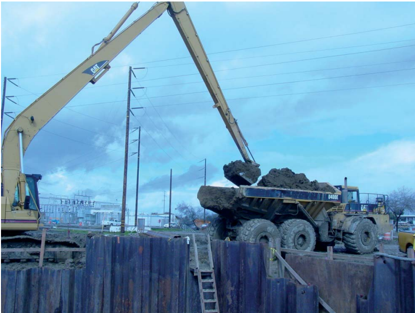
FIGURE 5.24 Equipment surcharge load on an excavation.
