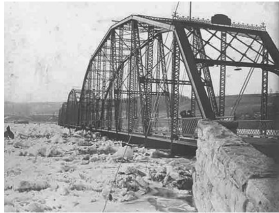
Figure 4.7 Susquehanna river ice jam and flood which destroyed the Catawissa Bridge in Pennsylvania, USA on 9 March 1904.
