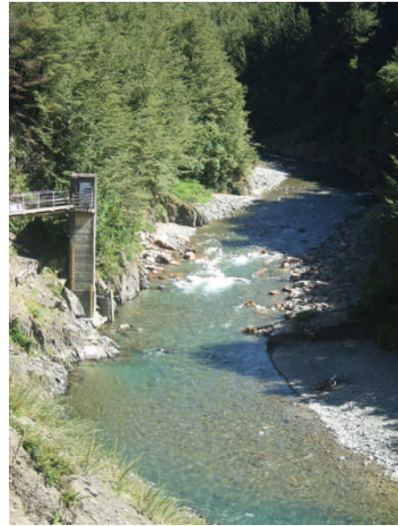
Figure 8.11 A stilling well in a large concrete tower beside a mountain river. In this case the tower has to be high to record high levels in large floods. Note the external staff gauge attached to the concrete tower.
